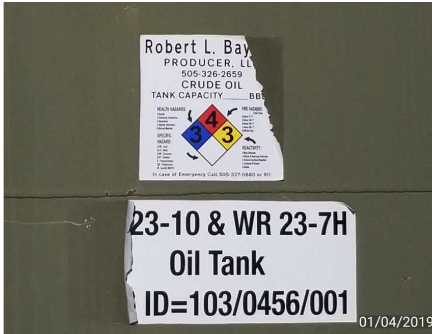
Photo 7. Tanks missing 400 bbl capacity on label.
