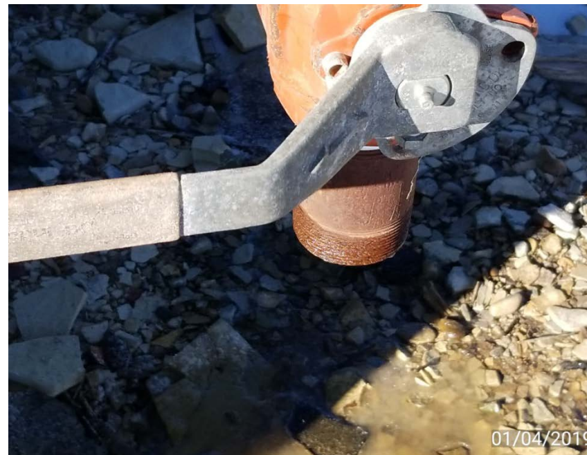
Photo 6. Separator valve leaking fluid on ground.
