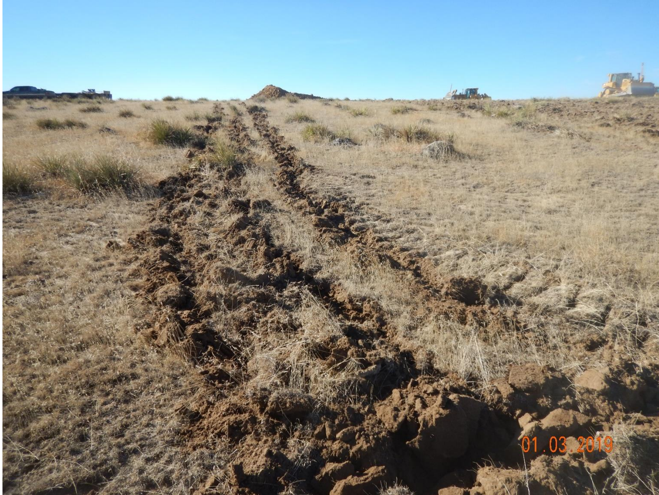
Photo 1: Photo taken from the southeast end of the location, facing west. Photo shows operator has installed surface roughening as a temporary stormwater BMP along perimeter prior to construction activities.
