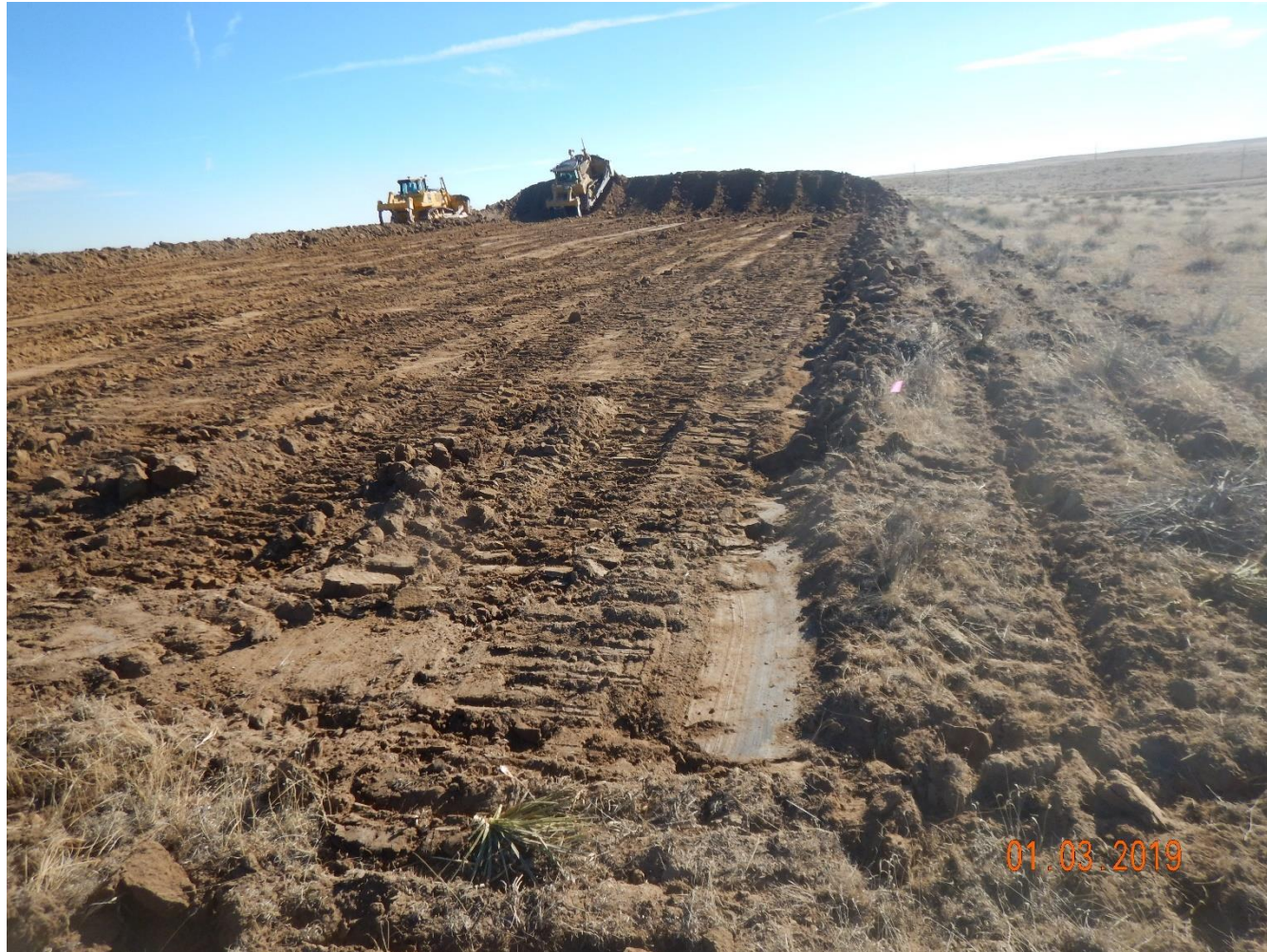
Photo 3: Photo taken from the north end of the location, facing west. Photo shows operator has installed surface roughening as a temporary stormwater BMP along perimeter prior to construction activities. Photo also shows topsoil salvage in process.
