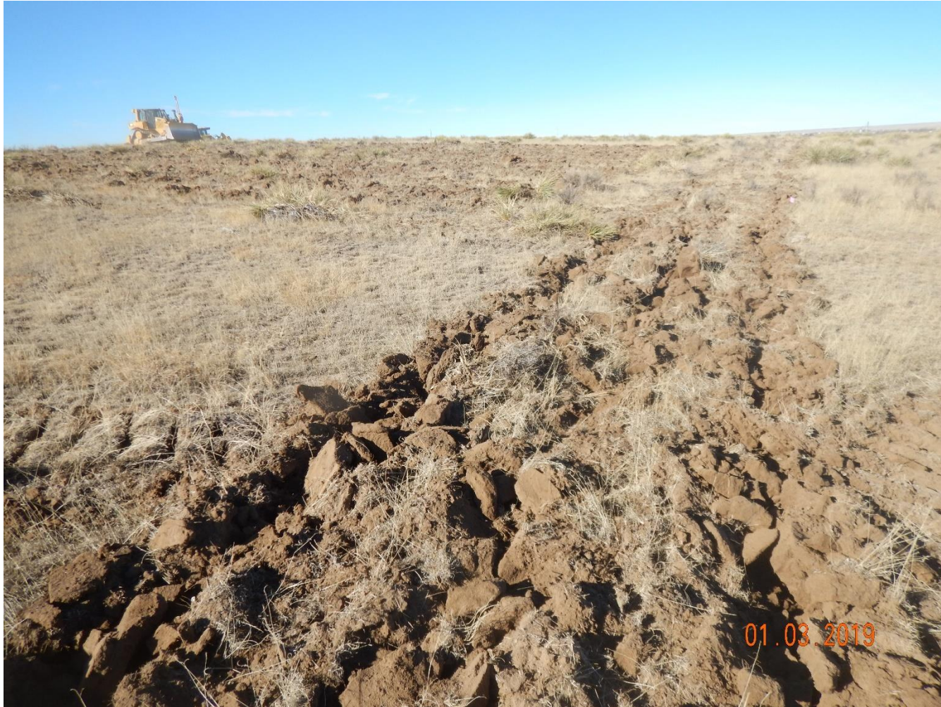
Photo 2: Photo taken from the southeast end of the location, facing north. Photo shows operator has installed surface roughening as a temporary stormwater BMP along perimeter prior to construction activities.
