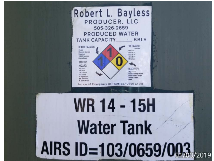
Photo 6. Tank missing capacity volume.
