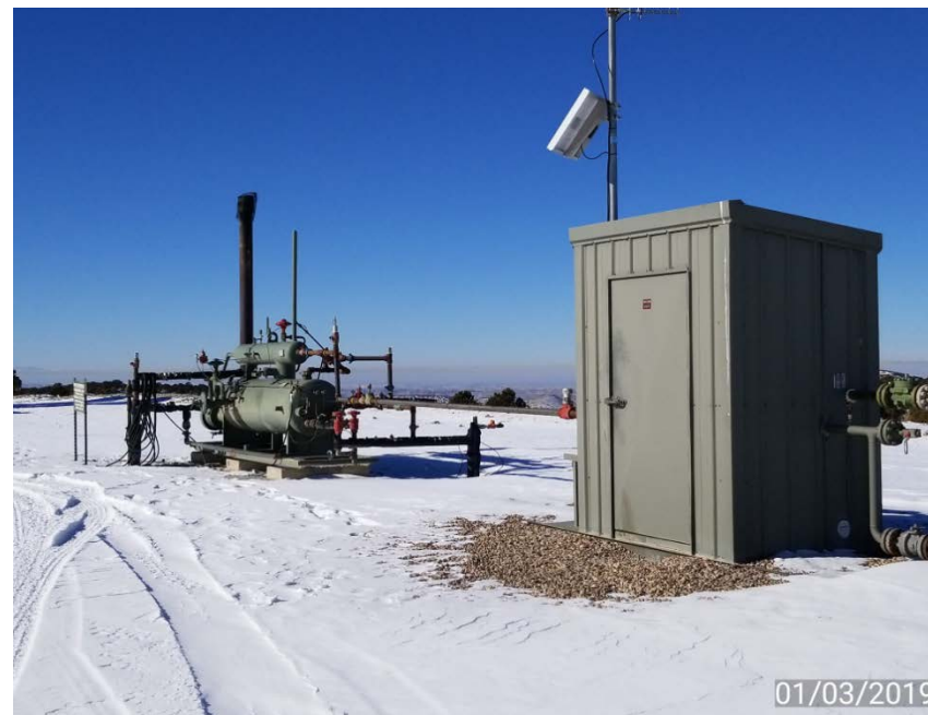
Photo 4. Gas meter building and separator.
