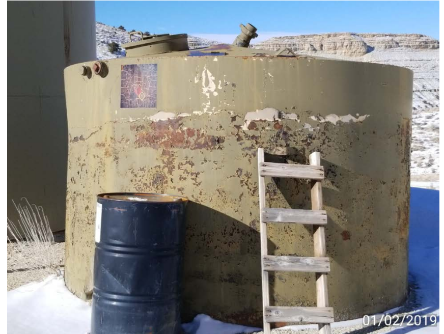
Photo 2. Tank that appears to be unused without complete labeling.
