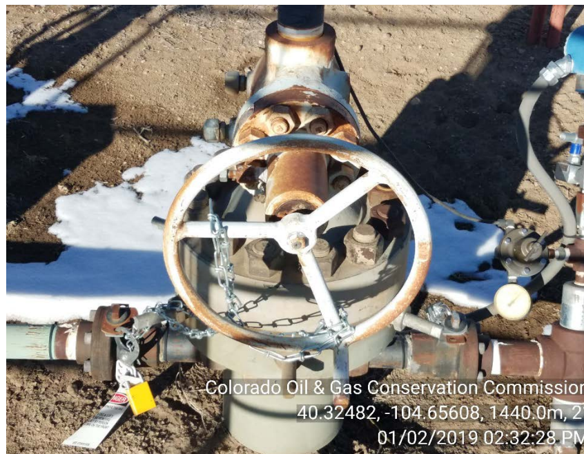
Wellhead master valve
