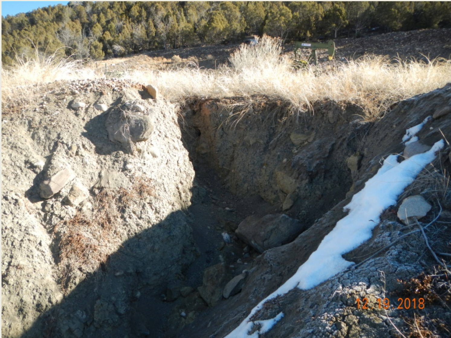
Photo 2. View of an erosional channel approximately 6 feet wide and deep within the western fill slope.
