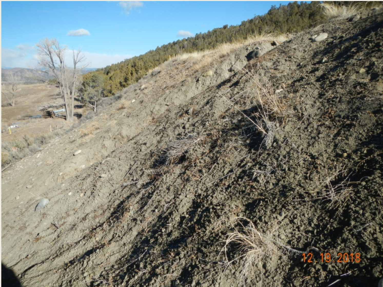
Photo 5. View of the western fill slope from the southwestern edge facing northward. Poor revegetation on fill slope.
