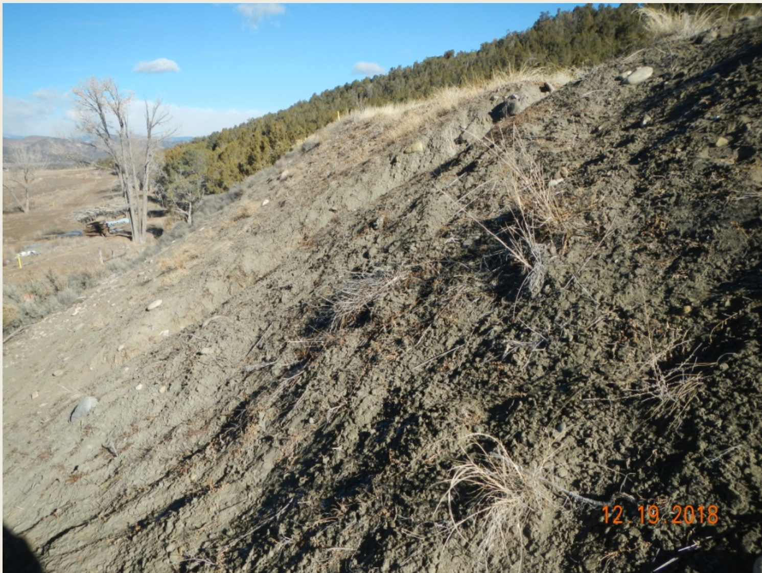
Photo 6. View of the western fill slope from the southwestern edge facing northward. Poor revegetation on fill slope.
