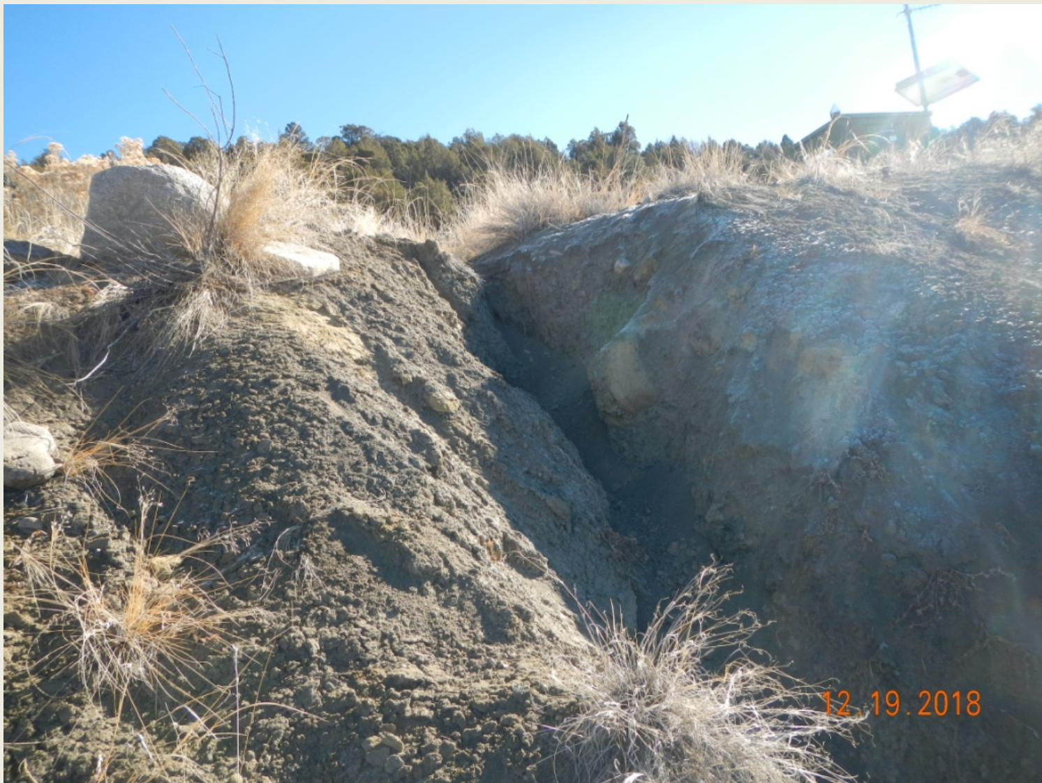
Photo 5. View of another erosional channel within the western fill slope approximately 4 feet wide and deep.
