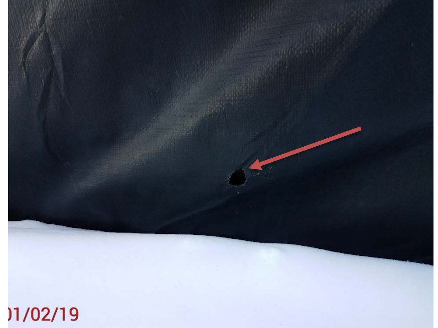
Location Photo #2, Hole in secondary containment liner.
