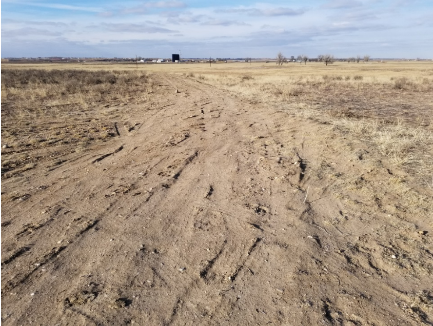
Photo 1. Photo taken from the access road, facing Northwest. Appears the Operator has not performed final reclamation activities. The equipment has been removed but the gravel still remains on the access road and location.
