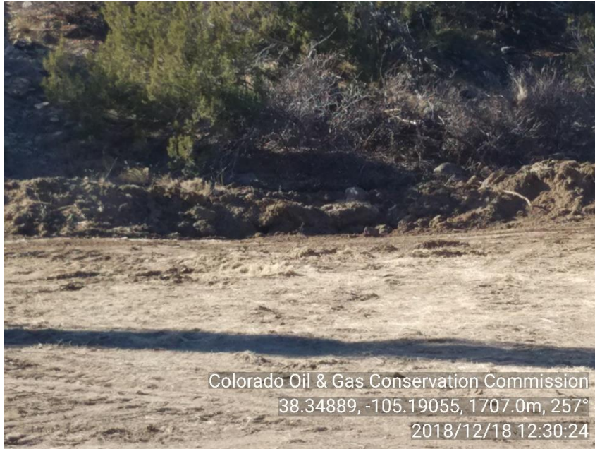
PHOTO 7: DITCH FOR STORM WATER DRAINAGE OF UP HILL SIDE OF LOCATION DOES NOT RUN CONTINUOUS ACROSS LOCATION
