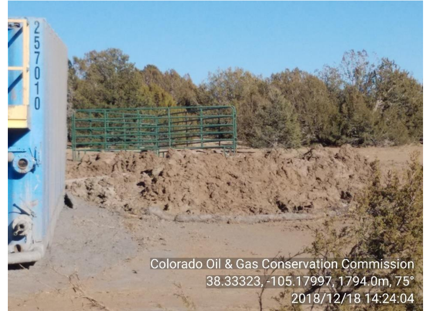
PHOTO 4: CUTTING TANK AND PILE OF MUD SET TO BE HAULED TO DISPOSAL
