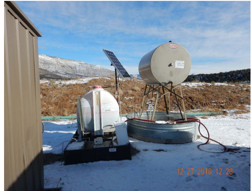
Photo #8 – Chemical storage tanks with secondary containment devices located south of tank battery.
