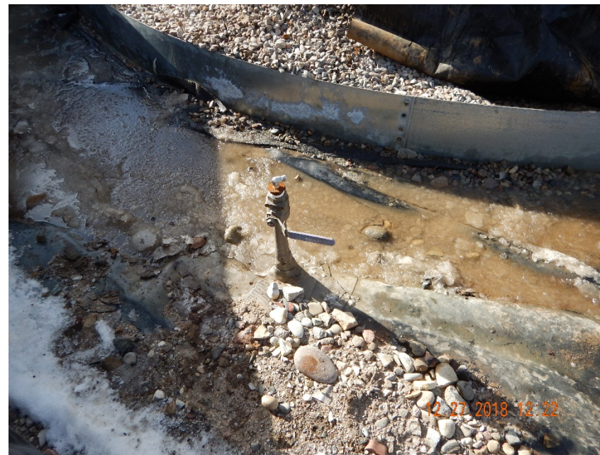
Photo #4 – 1" flowline riser protruding through liner at south end of tank battery.
