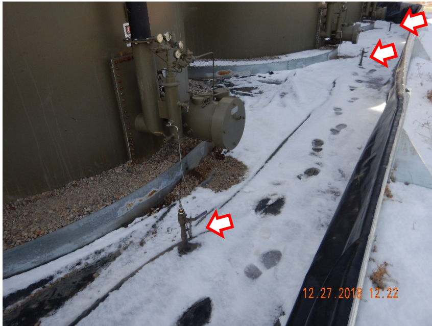
Photo #5 – Additional 1" flowline risers protruding through liner along east side of tank battery.
