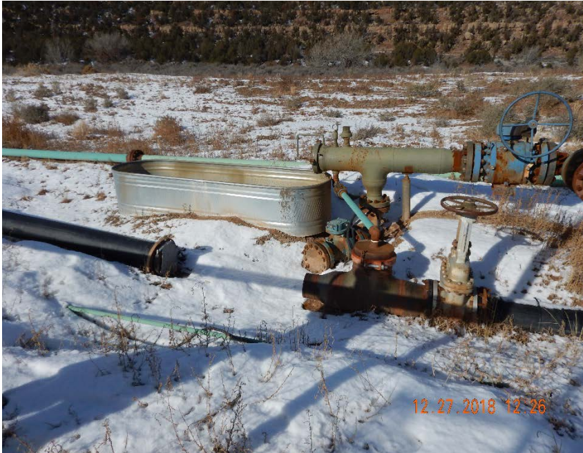
Photo #15 – Pig station and surface flowlines located north of crude oil/produced water tank battery.
