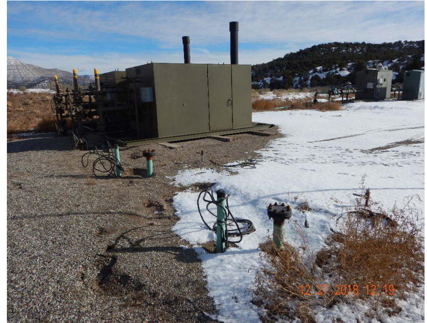
Photo #14 – Unused flowline risers observed west of separators.
