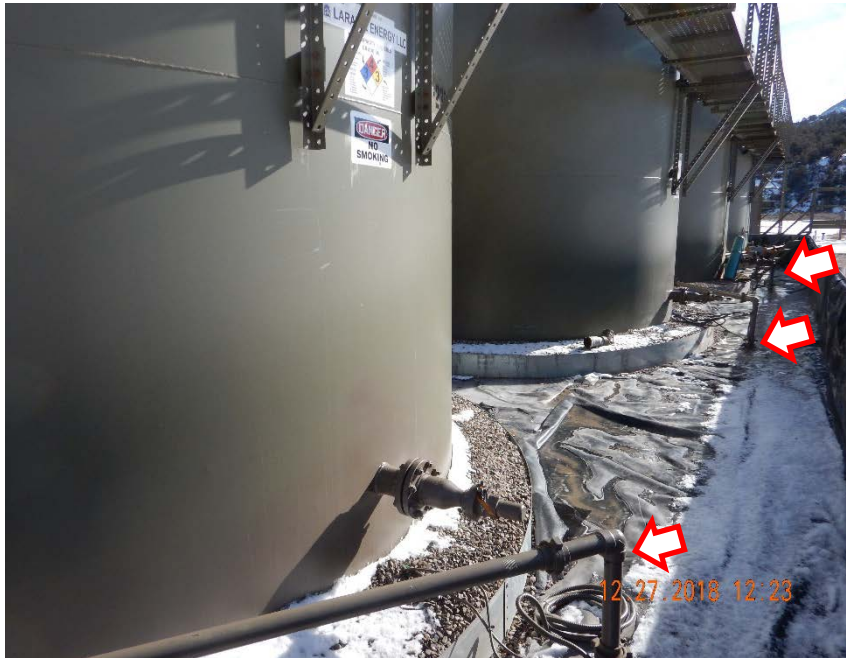
Photo #7 – 2" Flowline risers protruding through liner on west side of tank battery.
