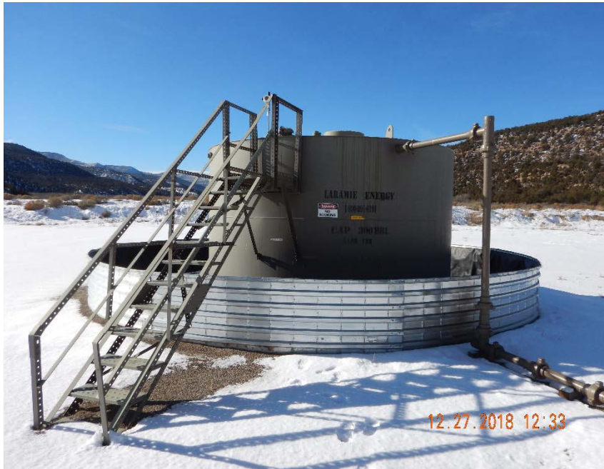
Photo #11 – 300 bbl sand tank inside of metal SPCC, located west of wellheads.
