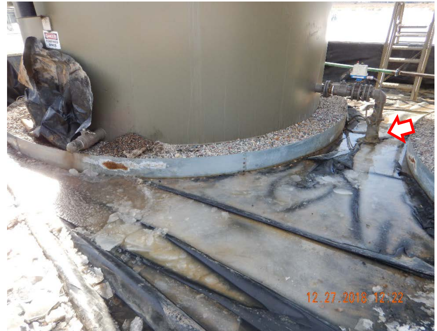
Photo #6 – Flowline riser and electrical conduit protruding through liner north of produced water AST. Note: other ASTs in tank battery had the same flowline configuration.
