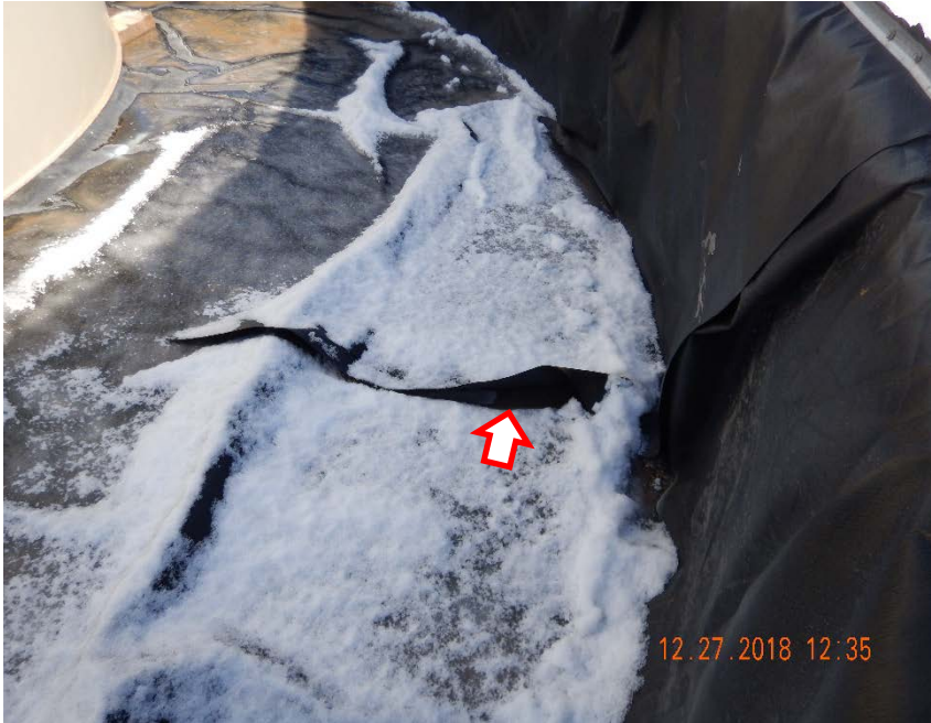
Photo #13 – Gap observed between liner panels inside southeast corner of sand tank SPCC.
