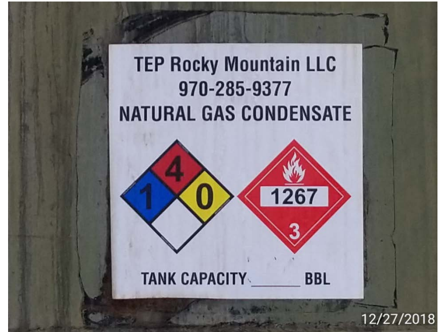
Photo 2. Tank without 300 BBL capacity label.
