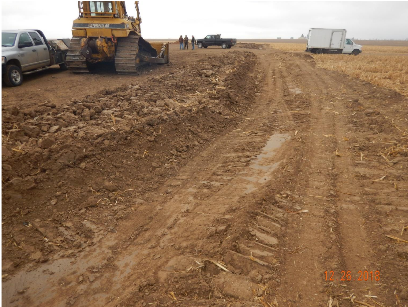
Photo 8: Photo taken from the southeast corner of the location, facing north. Photo shows a sotrmwater ditch has been constructed along the perimeter of the pad.
