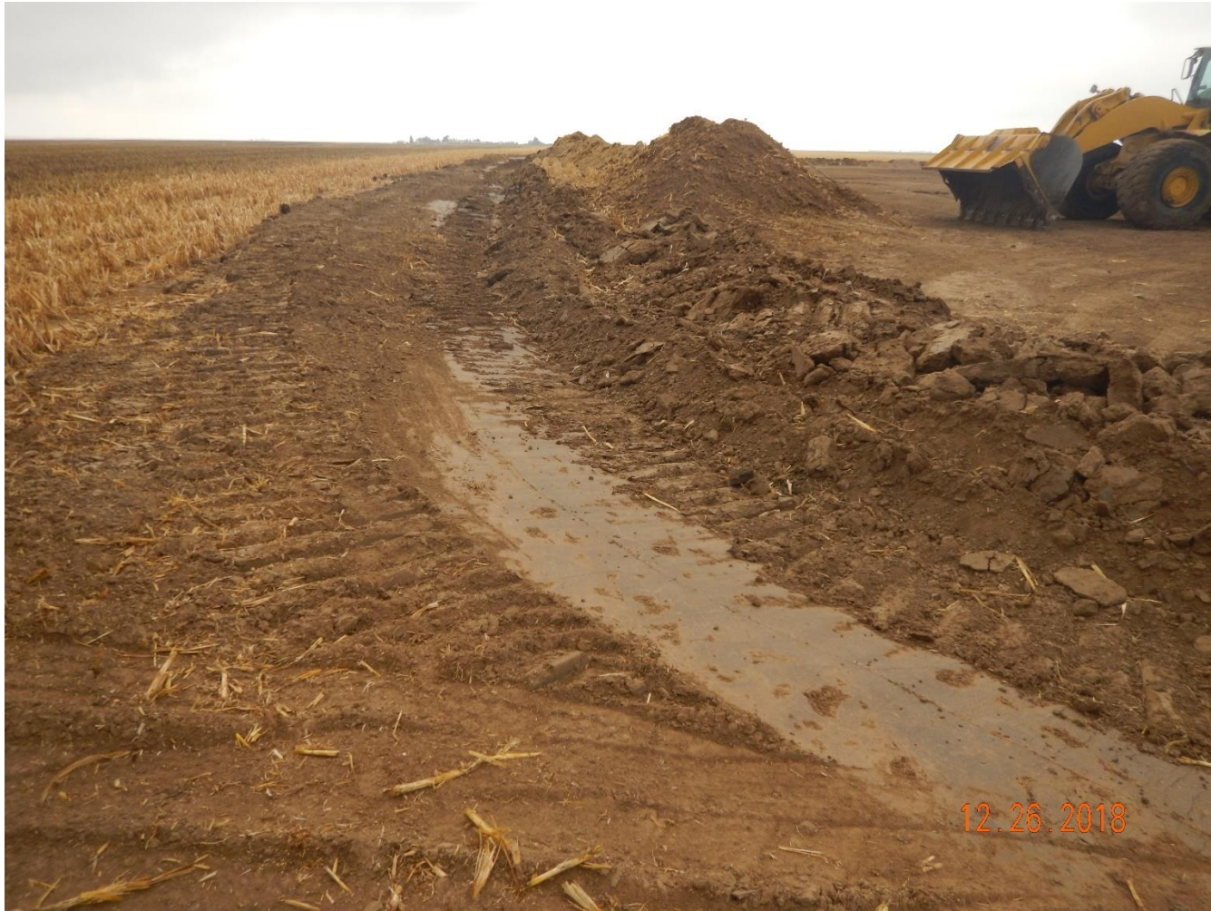
Photo 7: Photo taken from the southeast corner of the location, facing west. Photo shows a sotrmwater ditch has been constructed along the perimeter of the pad.
