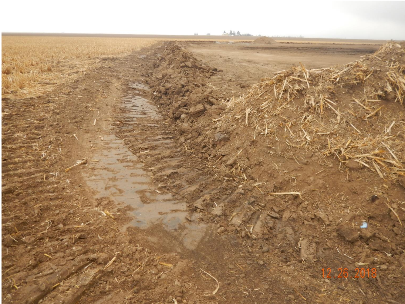
Photo 5: Photo taken from the southwest corner of the location, facing north. Photo shows a sotrmwater ditch has been constructed along the perimeter of the pad.
