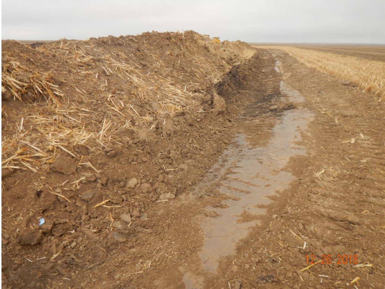
Photo 6: Photo taken from the southwest corner of the location, facing east. Photo shows a sotrmwater ditch has been constructed along the perimeter of the pad.
