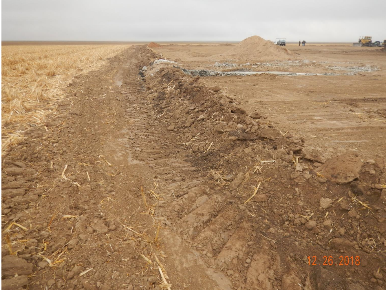
Photo 3: Photo taken from the northwest corner of the location, facing east. Photo shows a sotrmwater ditch has been constructed along the perimeter of the pad.
