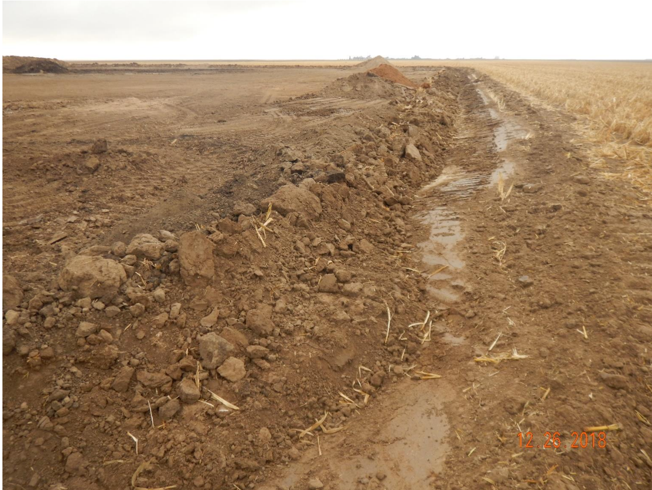
Photo 2: Photo taken from the northeast corner of the location, facing west. Photo shows a sotrmwater ditch has been constructed along the perimeter of the pad.
