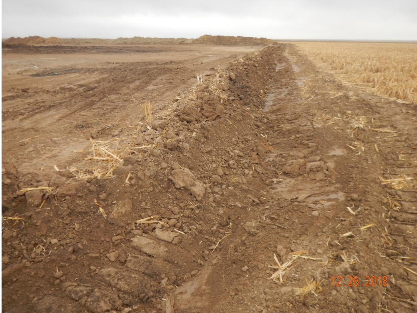
Photo 4: Photo taken from the northwest corner of the location, facing south. Photo shows a sotrmwater ditch has been constructed along the perimeter of the pad.
