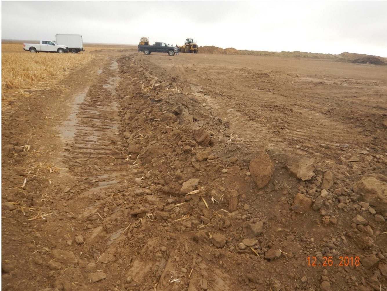
Photo 1: Photo taken from the northeast corner of the location, facing south. Photo shows a sotrmwater ditch has been constructed along the perimeter of the pad.
