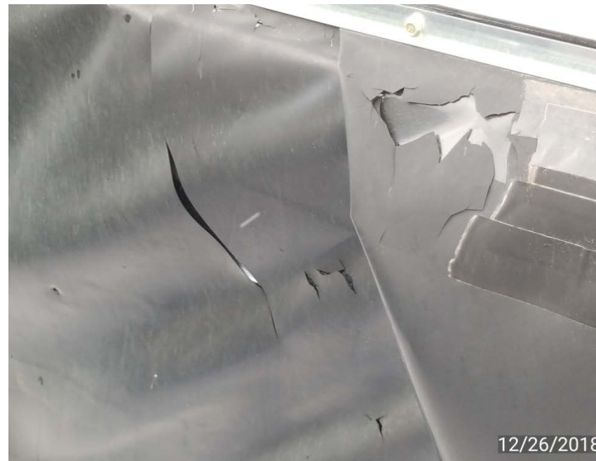
Photo 2. Tank secondary containment liner is damaged.
