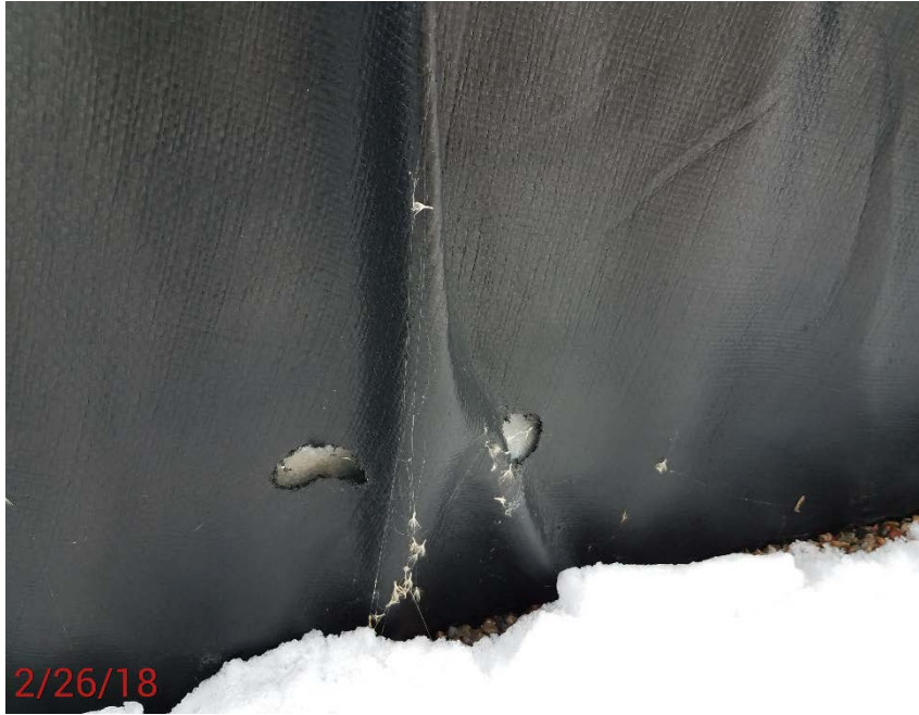
Location Photo #3, Holes in secondary containment liner.
