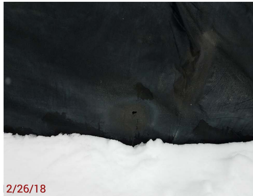
Location Photo #2, Hole in secondary containment liner.
