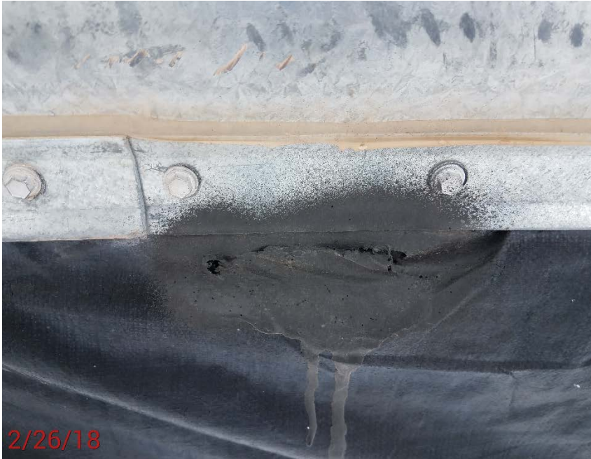
Location Photo #3, Hole in secondary containment liner.
