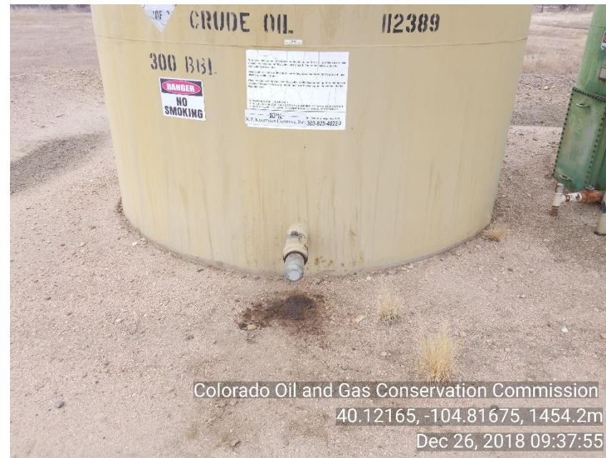
Photo 10 Stained soil crude oil tank
