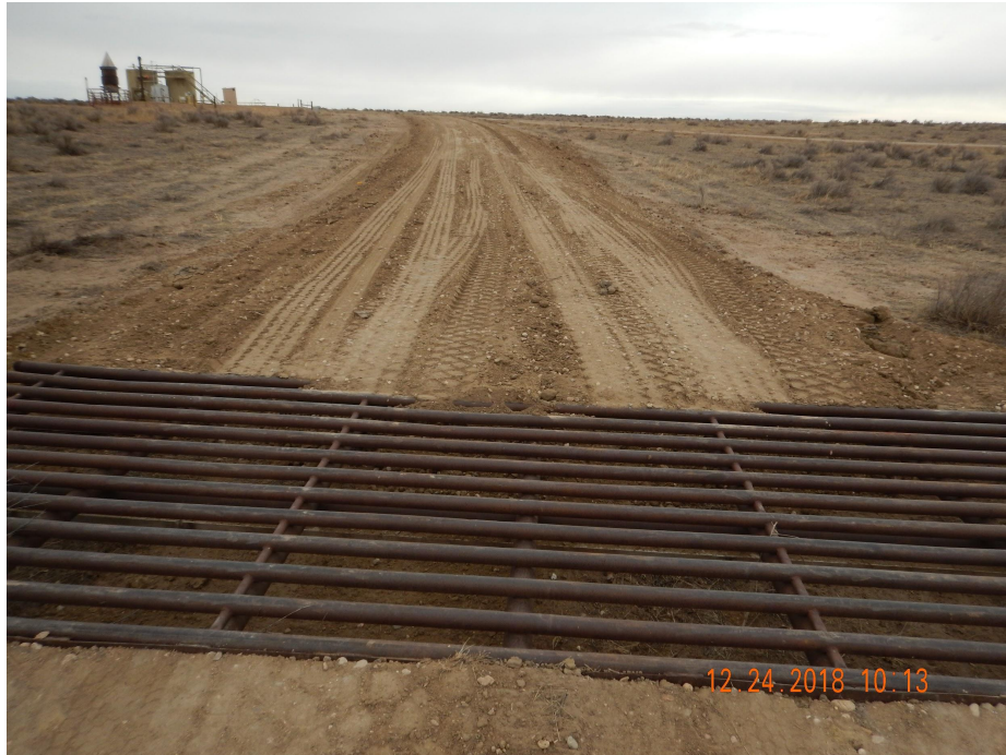
Photo 1. Photo taken from the northeastern entrance to location, facing East. Operator is in-process of stabilizing the access road. Cattle guard is likely intending to keep cattle out but may also serve as a vehicle tracking device BMP.
