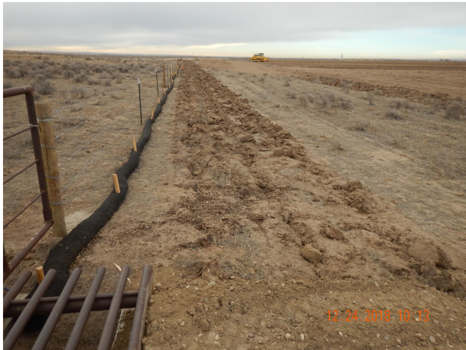
Photo 3. Photo taken from the northeastern entrance to the location, facing South. Operator has installed temporary stormwater BMPs (surface roughening and filtrex wattles) around the entire perimeter of the location during construction operations.
