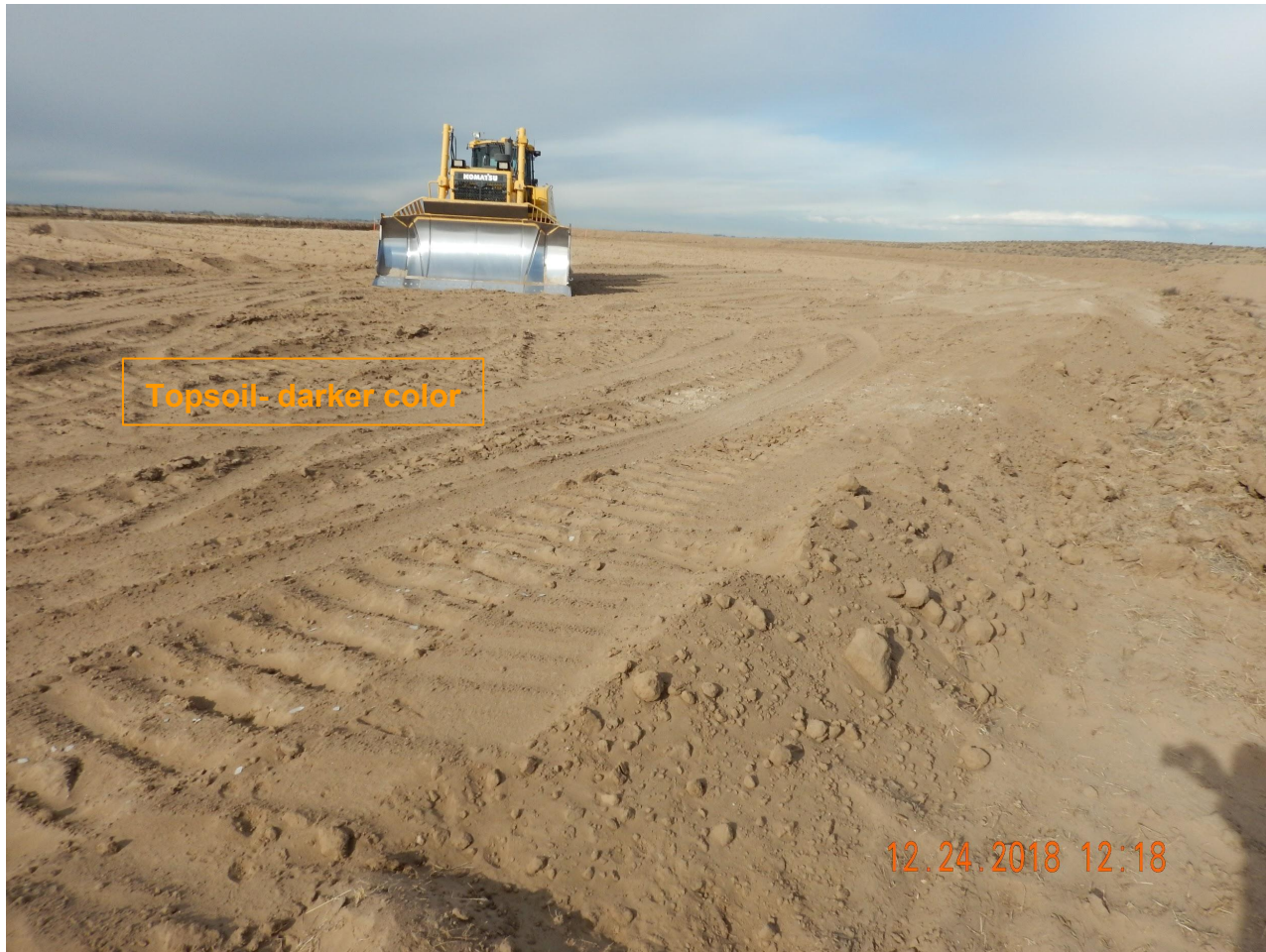
Photo 15. Photo taken from the southeastern well pad area, facing North. Appears topsoil is being used as fill material.
