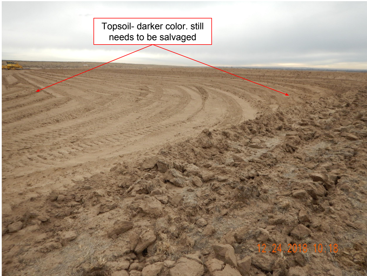
Photo 7. Photo taken from the southwestern perimeter of the location, facing Southeast. Photo illustrates topsoil that still needs to be salvaged from the southern well pad area.
