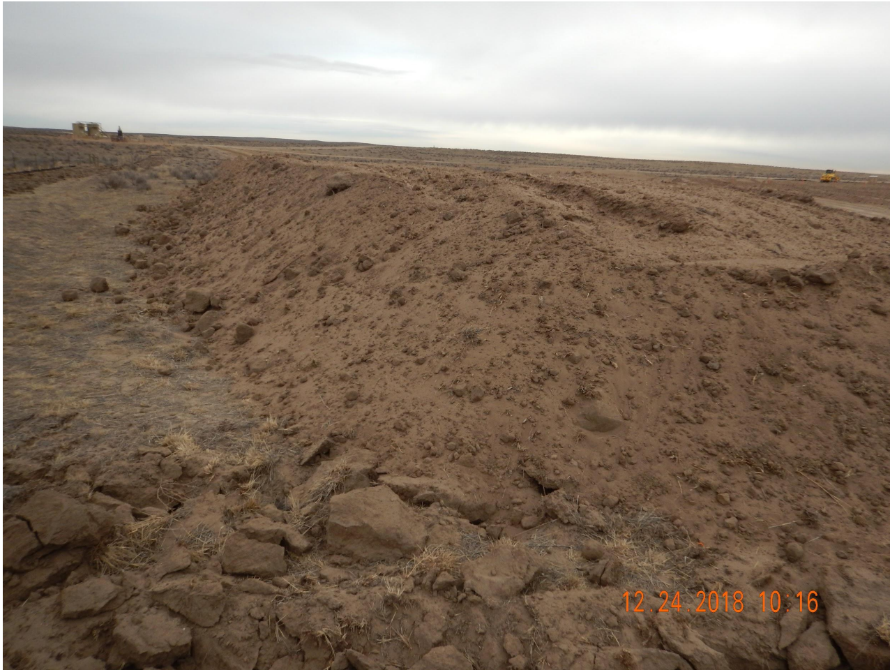
Photo 5. Photo taken from the northwest perimeter of the location, facing East. Photo illustrates the topsoil stockpile that shall be stabilized from wind and water erosion and protected from weed establishment.
