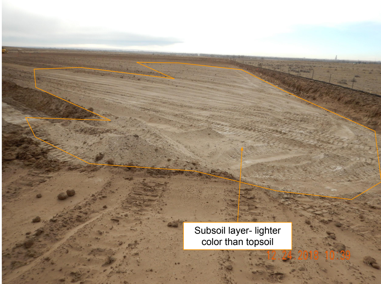
Photo 14. Photo taken from the northwestern well pad area, facing South. Photo further demonstrates the subsoil layer which is differentiated from the darker topsoil layer. An approximate area is shown above where the Operator has salvaged off topsoil.
