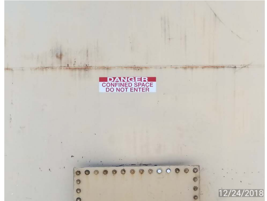
Photo 2. 90 bbl tank without required labels.
