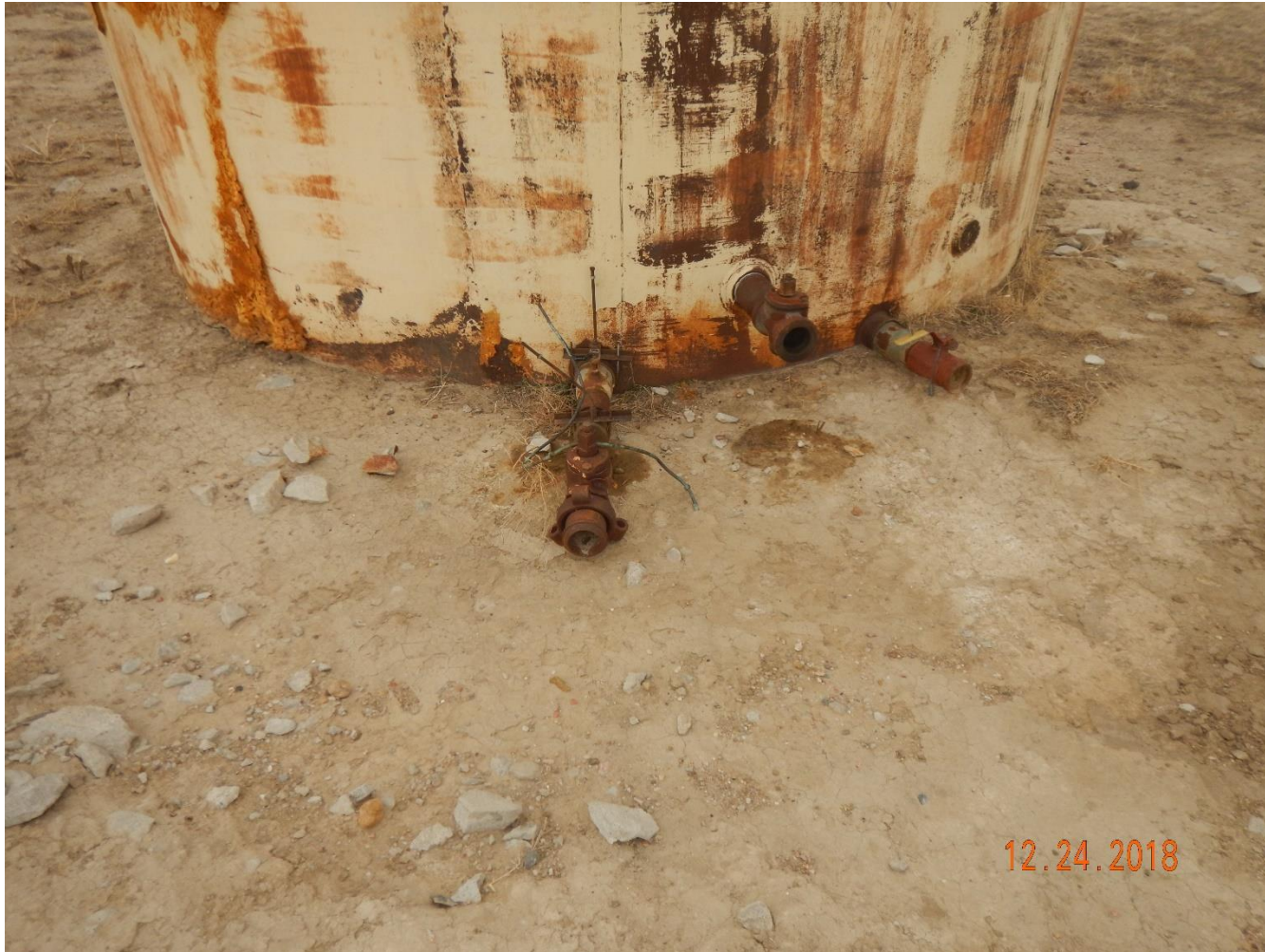
Photo 7: Continued from photo 6. Photo shows contaminated soil due to chemical discharge from the tanks have not been cleaned or removed.
