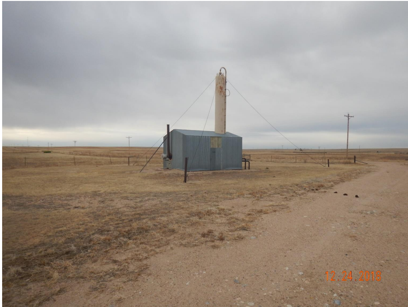
Photo 1: Photo taken from the south end of location, facing southwest. Previous inspections required operator to conduct final reclamation. Photo shows that oil and gas facilities/equipment/trash debris remains on location. Photo also shows access road remains. Unable to find evidence that final reclamation has been conducted in accordance with 1004 rules and requirements.
