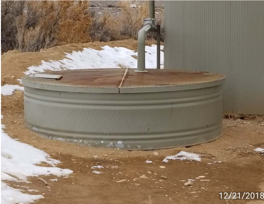
Photo 5. Tank missing labels.
