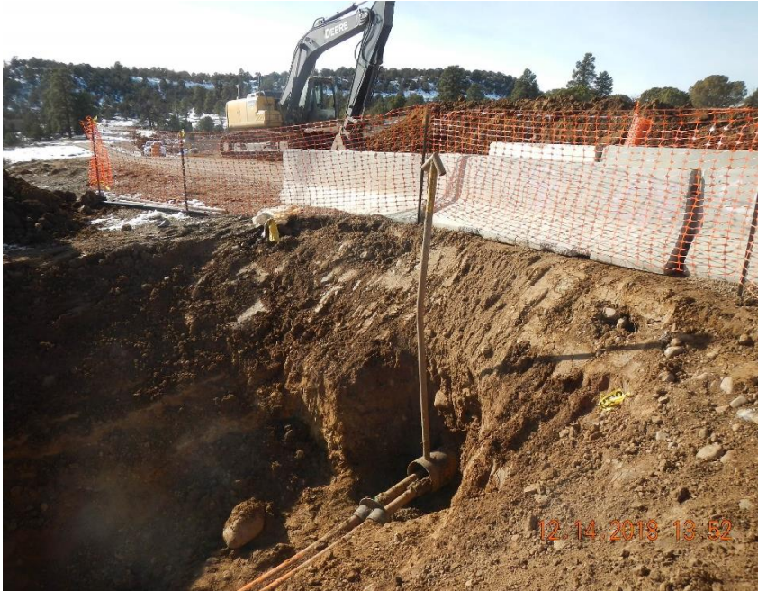
12" steel casing sleeve under access road.
