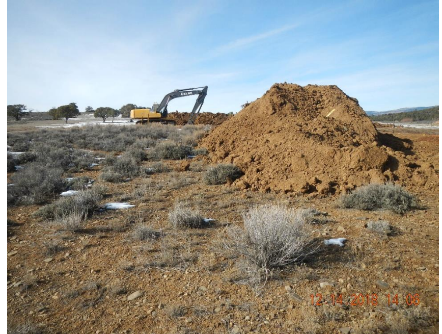
Impacted material excavated from east side of access road. Install BMPs to prevent migration of impacted material.
