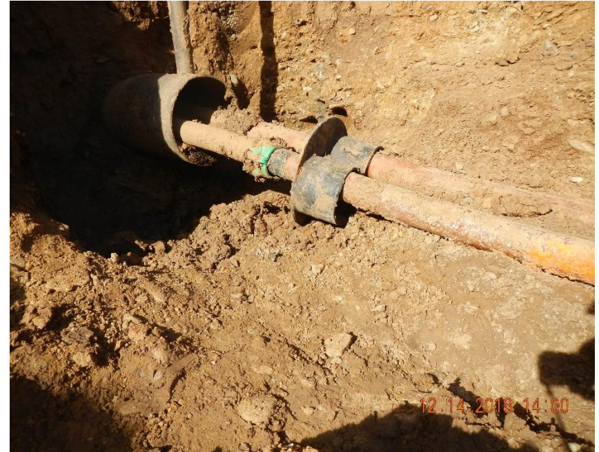
3" fiberglass pipelines along east side of access road.
