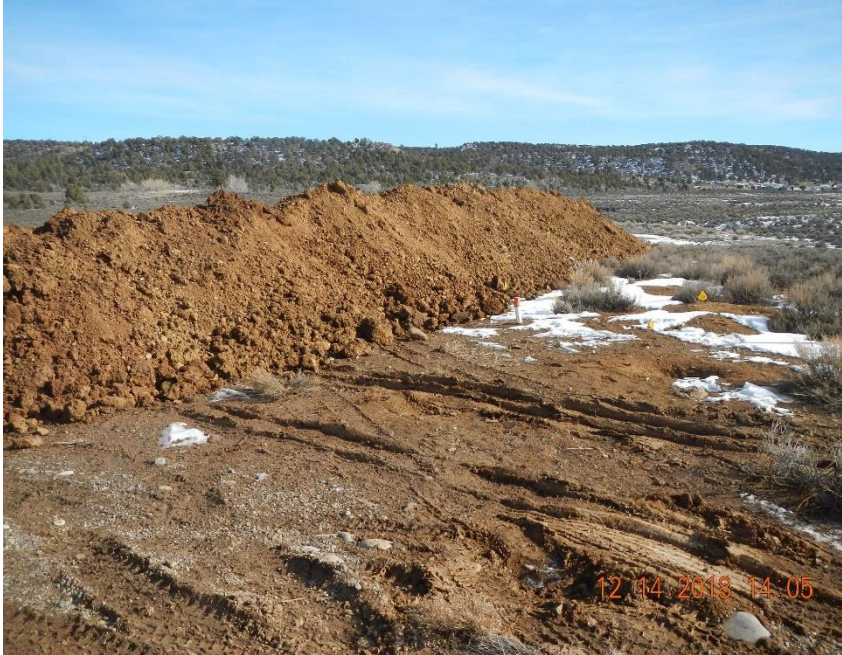
Excavated material along east side of access road. Install BMPs to prevent migration of impacted material.
