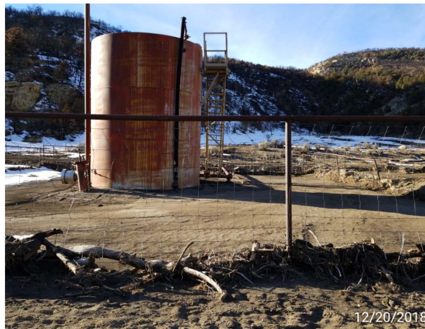
Photo 2. Tank berm on east is washed out.
