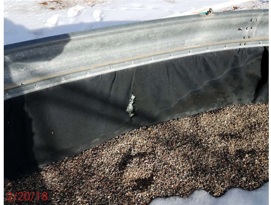
Location Photo #4, Holes in containment liner.
