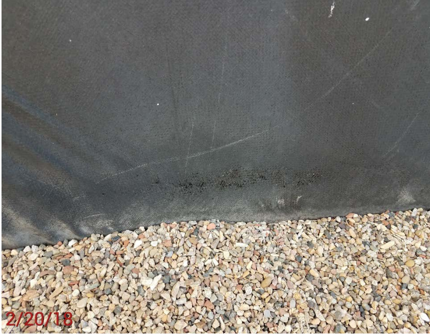
Location Photo #5, Holes in containment liner.
