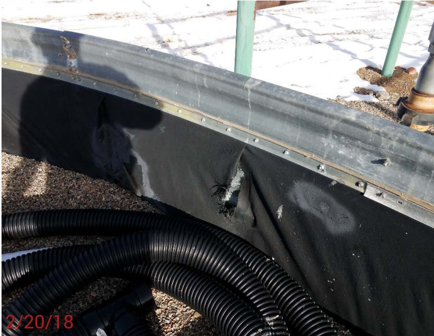
Location Photo #3, Holes in containment liner.
