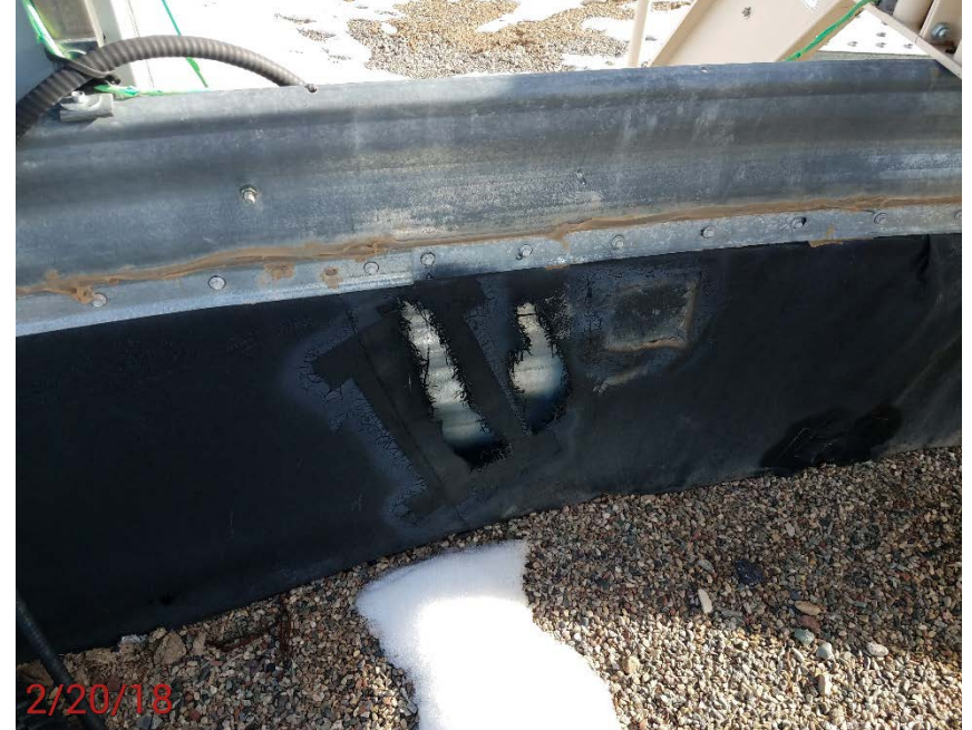
Location Photo #2, Holes in containment liner.
