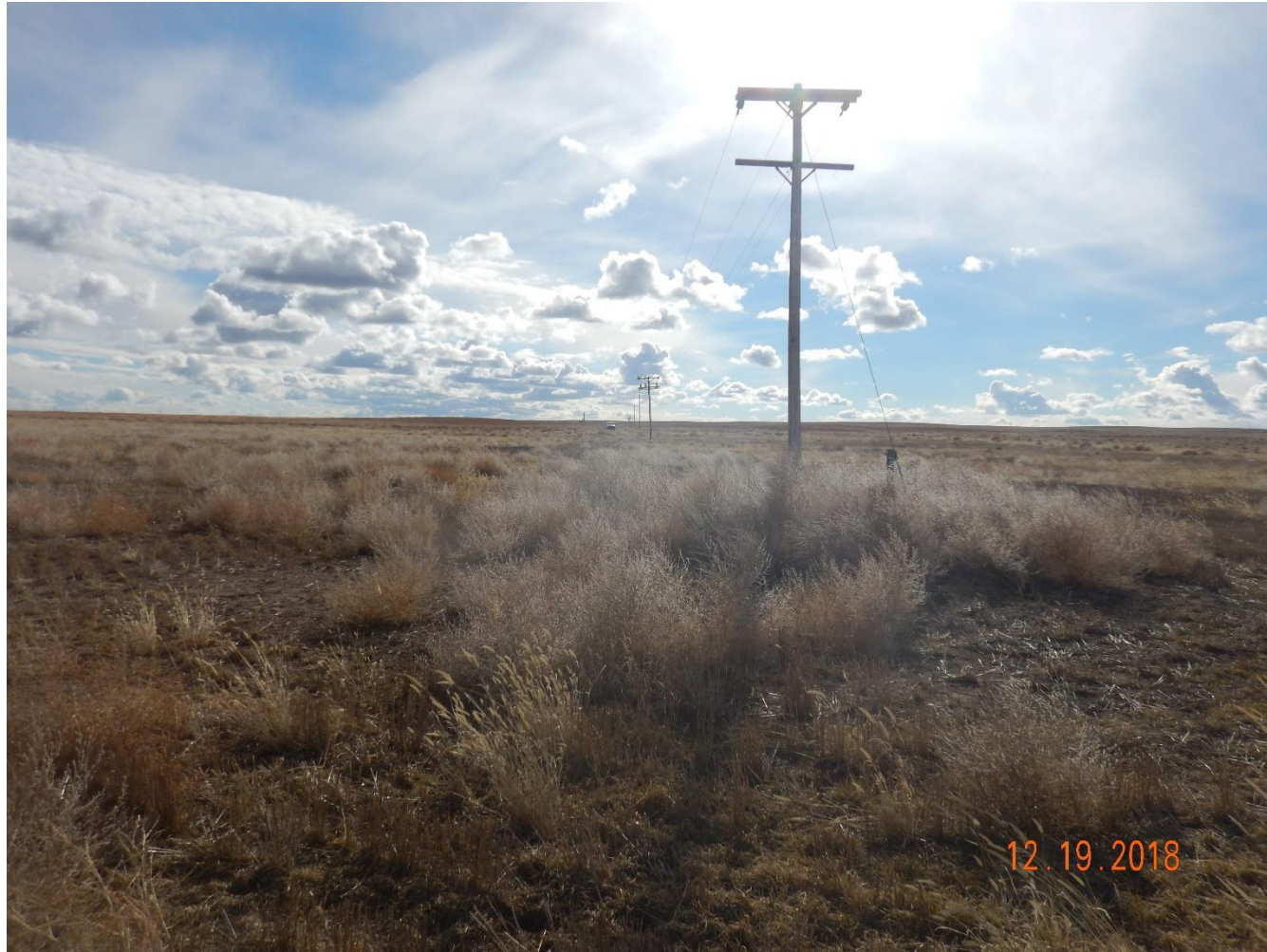
Photo 4: Photo taken from the well location, facing south. Photo shows utility power lines (4 poles) leading north from the Rudnik 33-27 ending at the Rudnik 32-27. This is surface equipment associated with the abandoned oil and gas location and requires removal.
