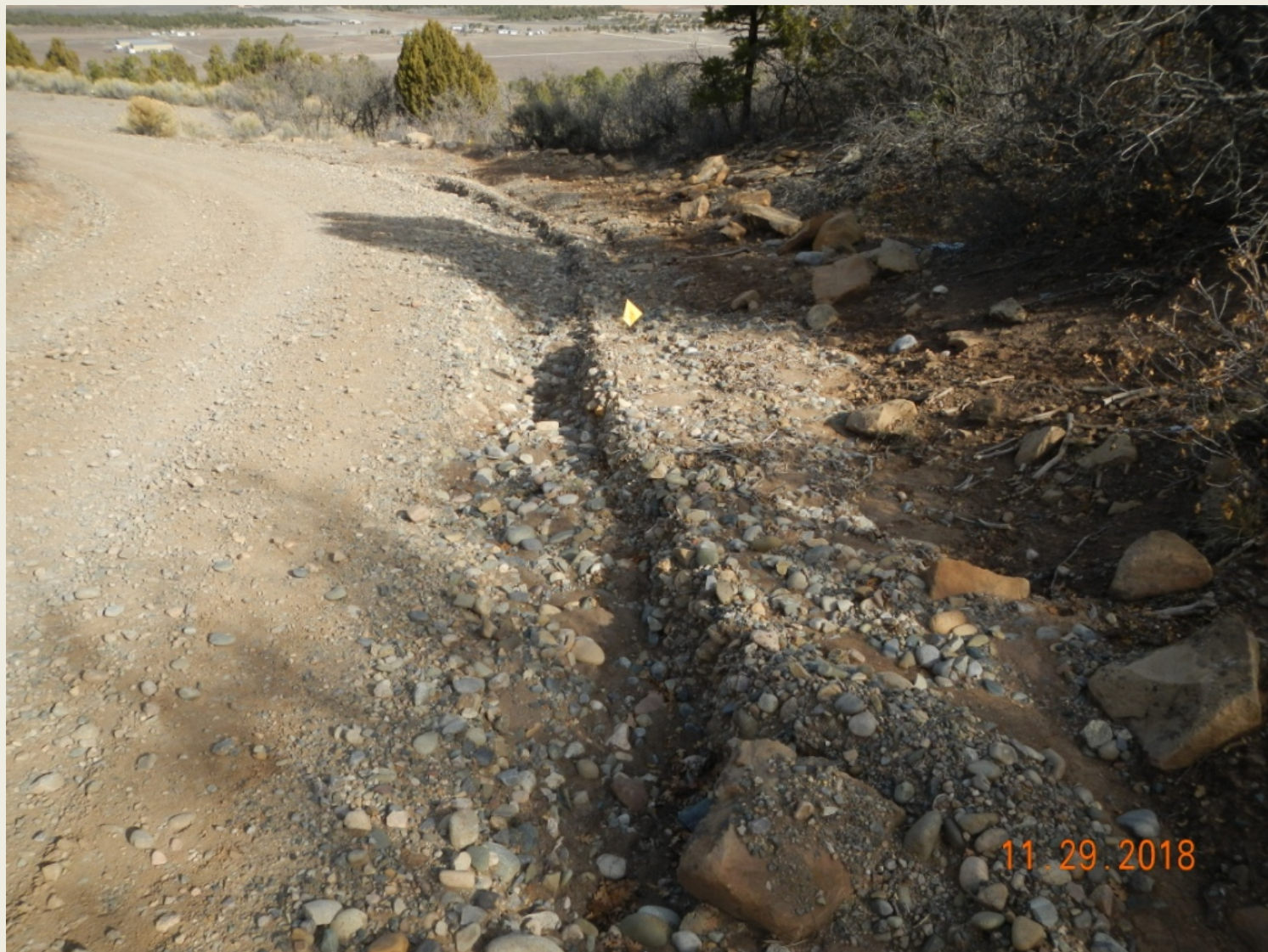
Photo 3. Another view of erosion occurring along the access road where rock and sediment transport and deposition is occurring.
