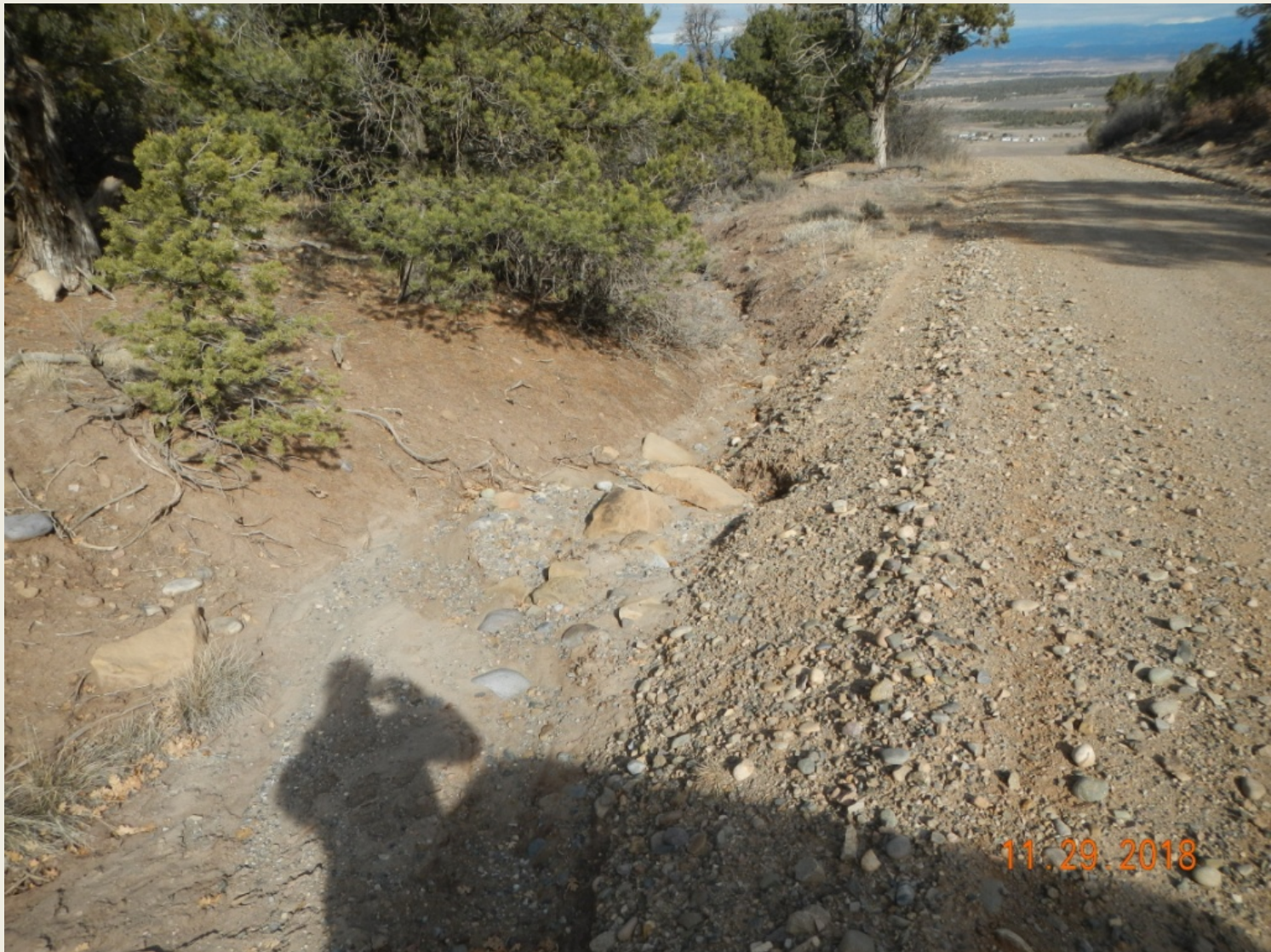
Photo 4. View of erosion occurring near the beginning of the access road. Stormwater controls are needed to stabilize erosional downcutting, and sediment transport.
