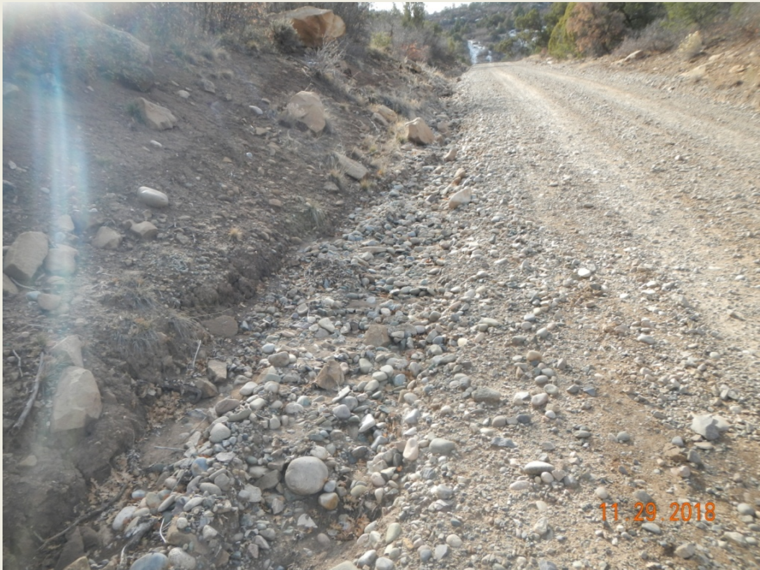
Photo 2. View of erosion occurring along the access road. Stormwater controls are needed.
