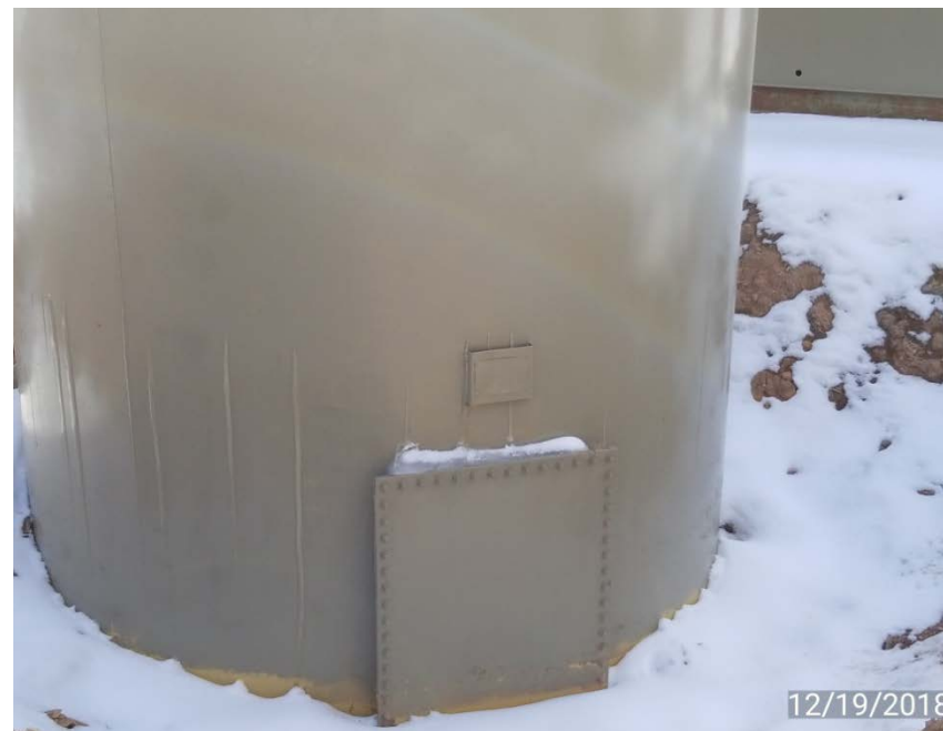
Photo 2. Tank without label for NFPA, capacity, and contents.
