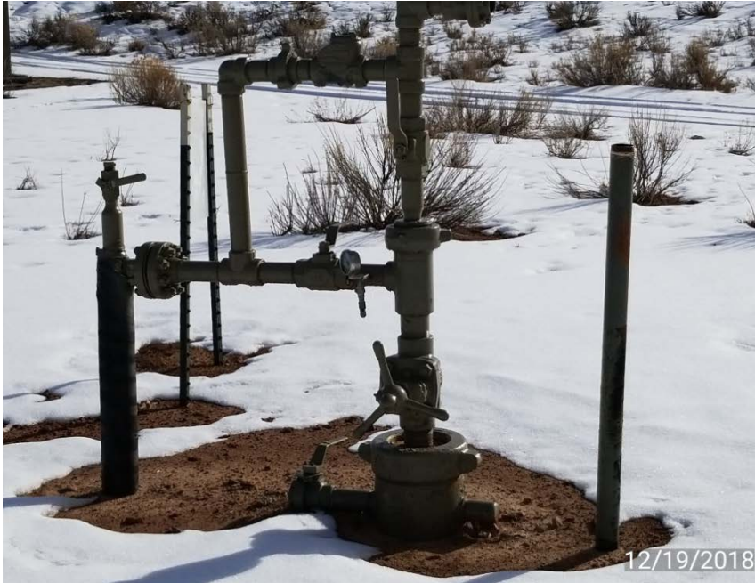
Photo 5. Riser next to well head not capped or locked out tagged out
