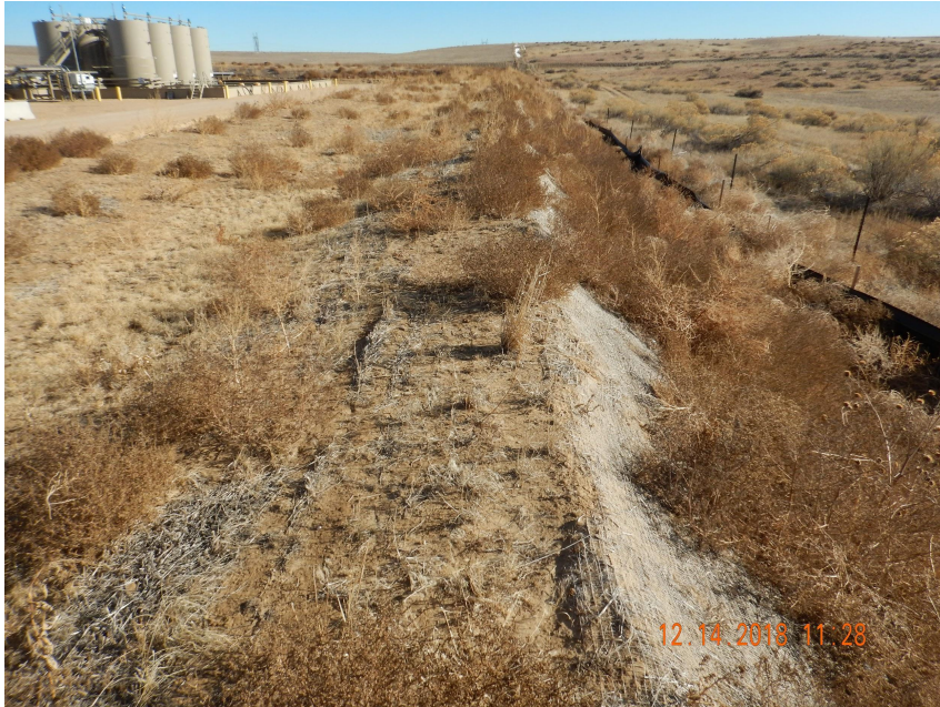
Photo 1. Photo taken from the southern southern topsoil stockpile, facing East. Operator has failed to prevent weed establishment on the topsoil stockpile. Note: Appears the Operator attempted to seed the topsoil with desirable vegetation (e.g., blue grama) but weedy, annual vegetation (Kochia) was observed throughout most of the stockpile fill slope areas. Note: Kochia was observed throughout cut and fill slopes of the well pad.
