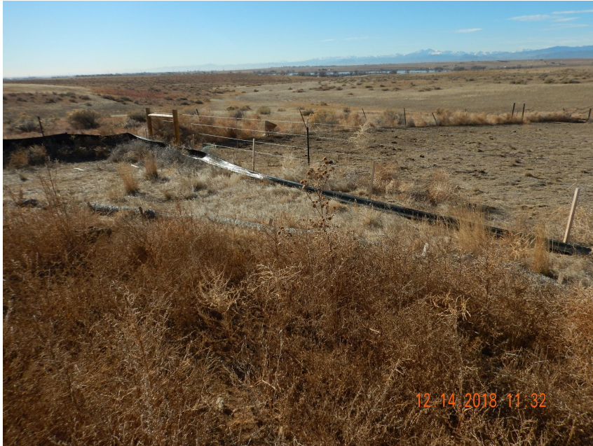
Photo 5. Photo taken from the southwestern perimeter of the location, facing Southwest. Silt fence BMP in need of maintenance.
