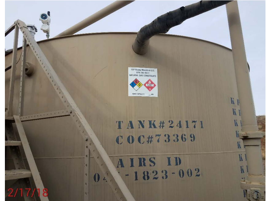
Location Photo #6, Missing tank capacity on all tanks.
