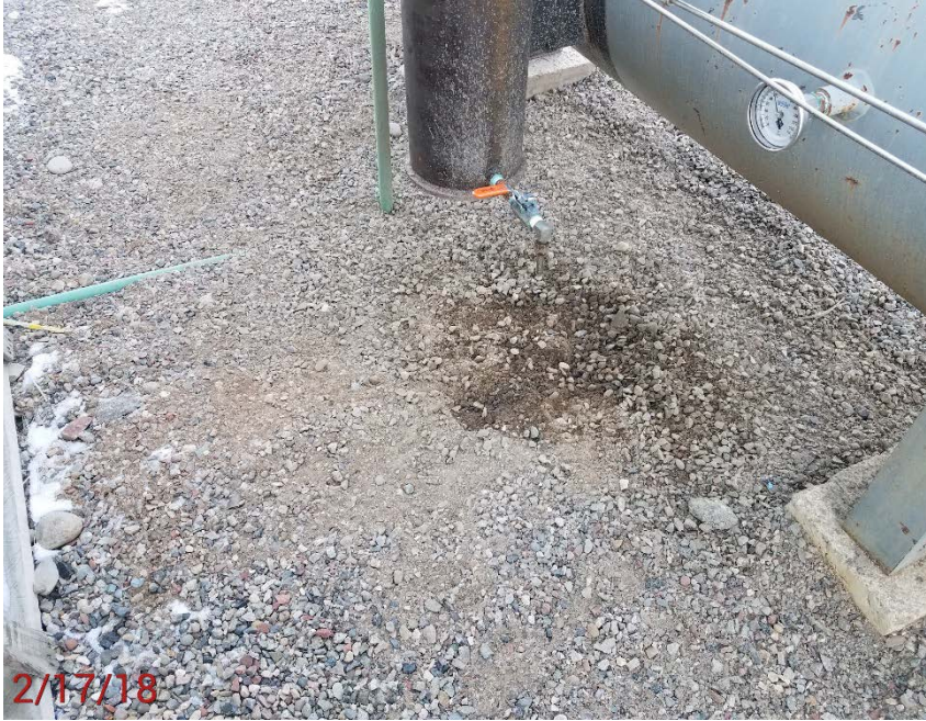
Location Photo #3, Stained soil next to the heater treater.
