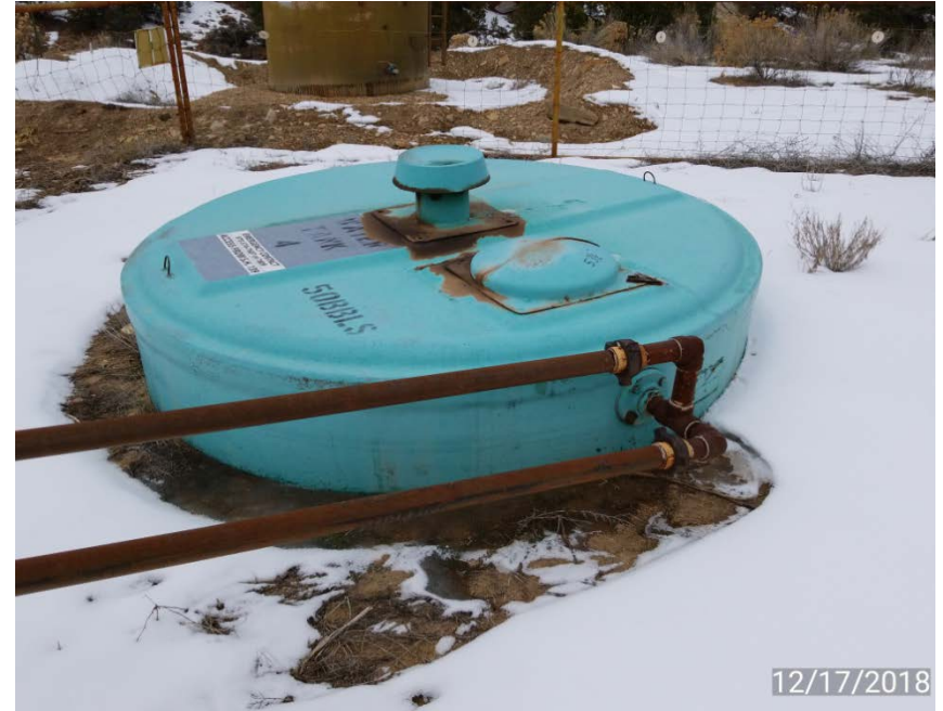
Photo 1. Tank without NFPA label.
