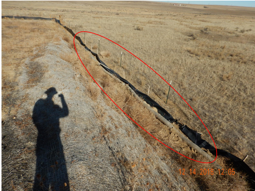
Photo 7. Photo taken from the north eastern topsoil stockpile, facing Northeast. Silt fence BMP in need of maintenance.
