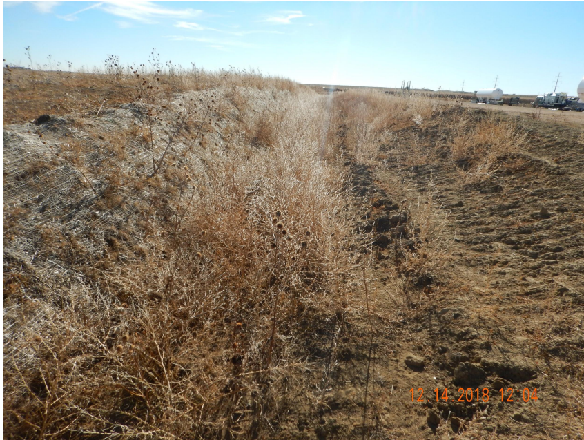
Photo 3. Photo taken from the north eastern topsoil stockpile, facing South. Operator has failed to prevent weed establishment on the topsoil stockpile. Note: Appears the Operator attempted to seed the topsoil with desirable vegetation (e.g., blue grama) but weedy, annual vegetation (Kochia) was observed throughout most of the stockpile.
