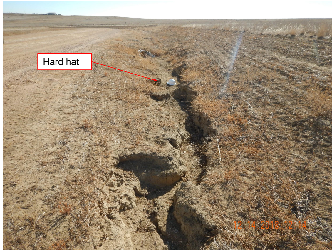
Photo 9. Photo taken along the access road just beyond the entrance of the location, facing South. Gully erosion has formed along a section of the access road.
