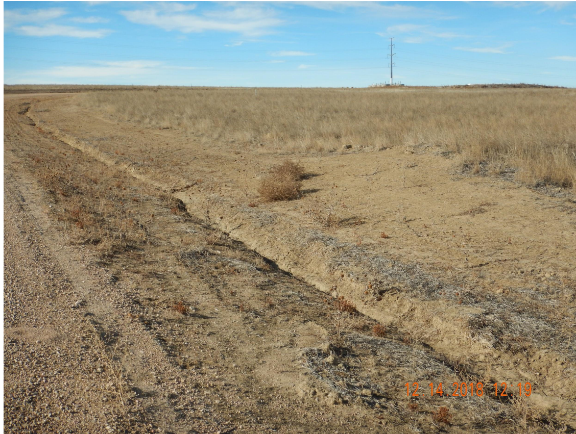
Photo 10. Photo taken from along the access road, facing West. Gully erosion is starting to form along the northern access road.
