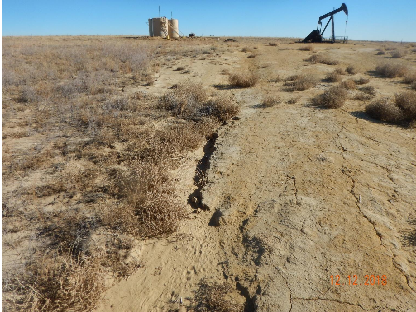
Photo 2: Photo taken from the North end of the location, facing south. Photo shows erosion has continued to degrade access road and location. Unable to find evidence of maintenance, or evidence that the required BMPs have been installed per 1002.f and corrective actions.
