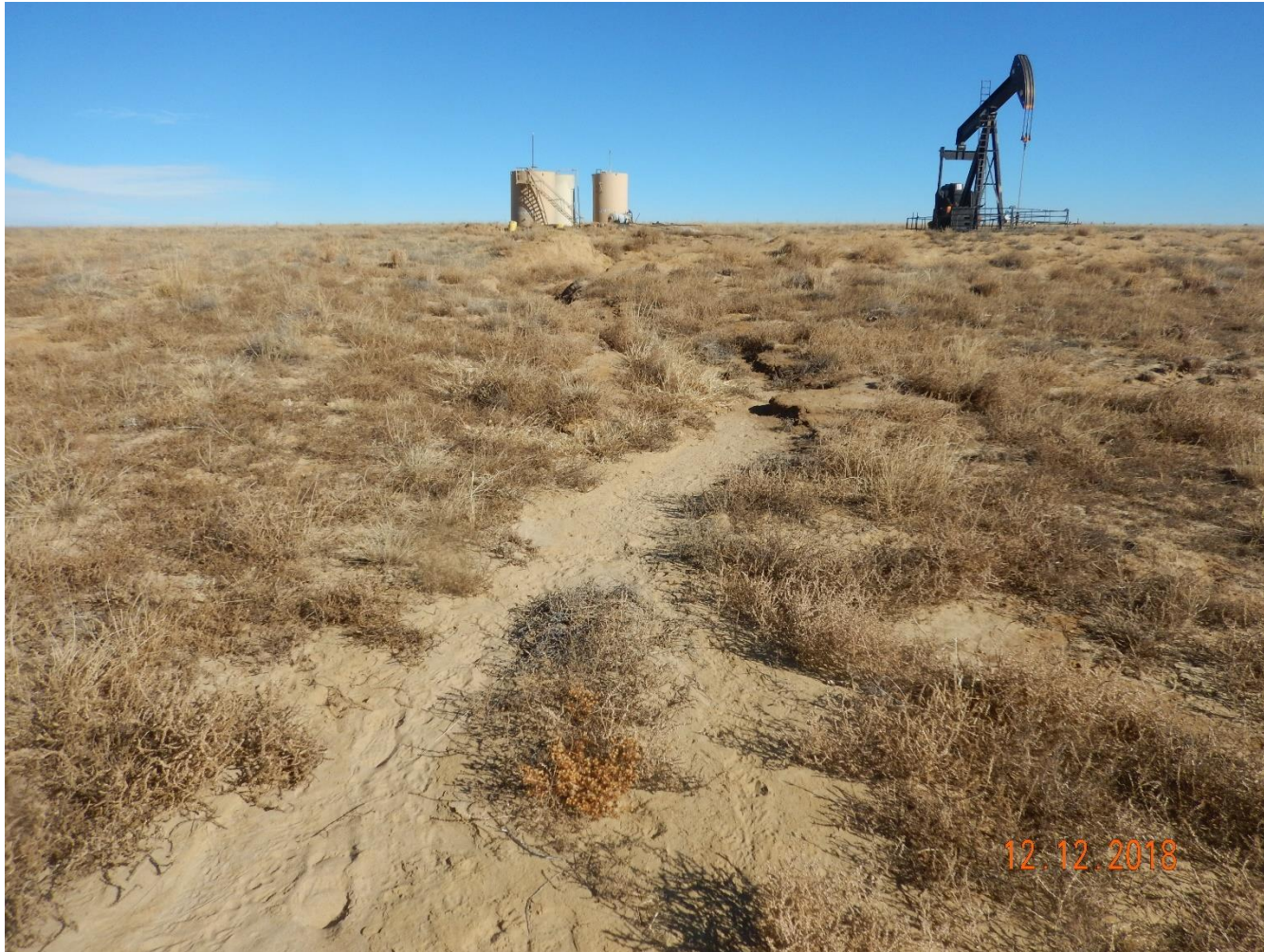
Photo 10: Photo taken from the interim areas west of the location, facing east. Photo shows stormwater erosion has been allowed to continue causing degradation to the location and interim areas. Unable to find evidence of maintenance and stabilization, or evidence that the required BMPs have been installed per 1002.f and per corrective actions.
