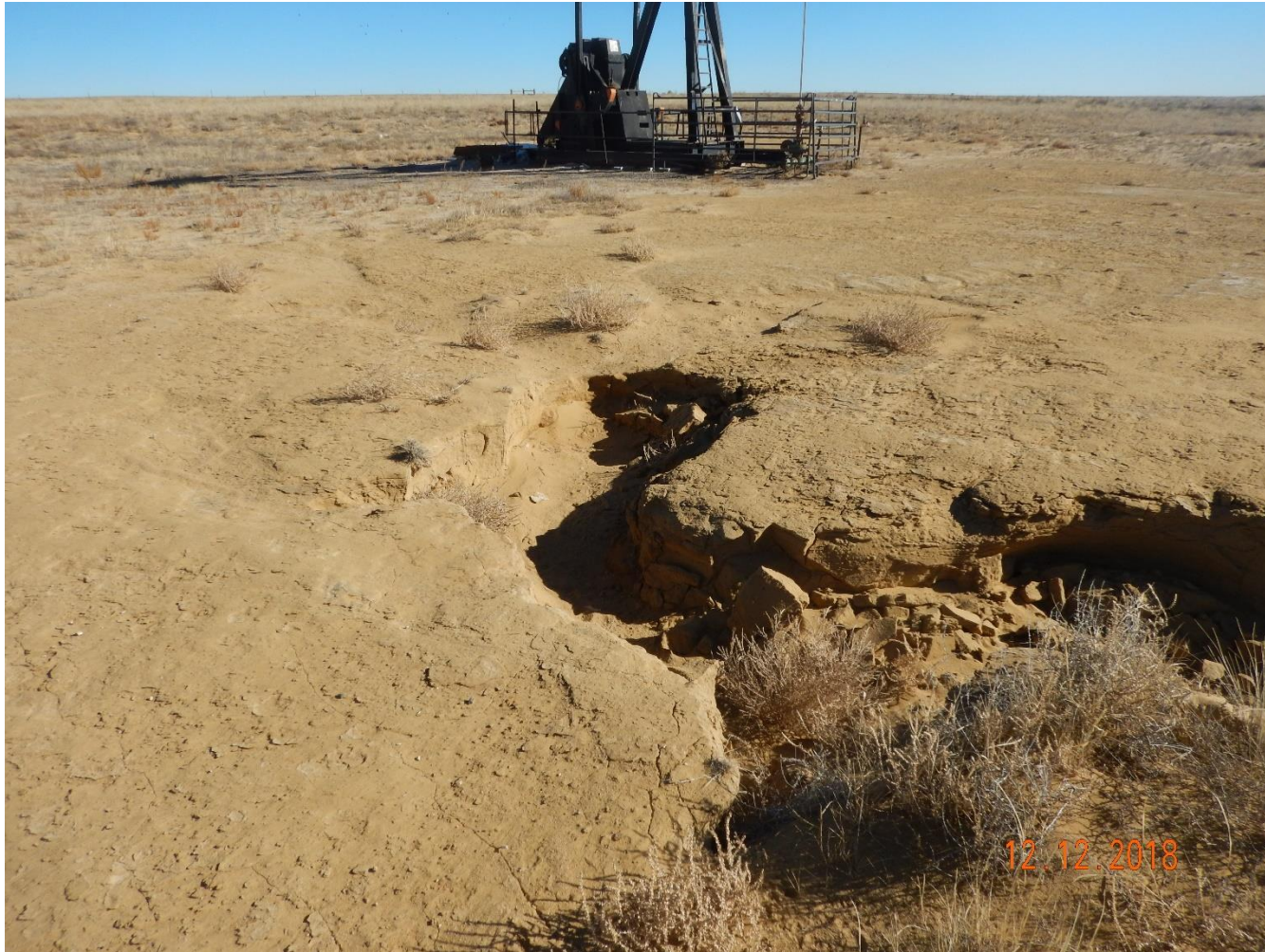
Photo 4: Photo taken from the northwest end of the production area, facing southeast. Stormwater erosion has created a large gully on the northwest end of the location. Photo shows the “head” of the erosion. Photo shows stormwater erosion has been allowed to continue causing degradation to the location and interim areas. Unable to find evidence of maintenance and stabilization, or evidence that the required BMPs have been installed per 1002.f and per corrective actions.
