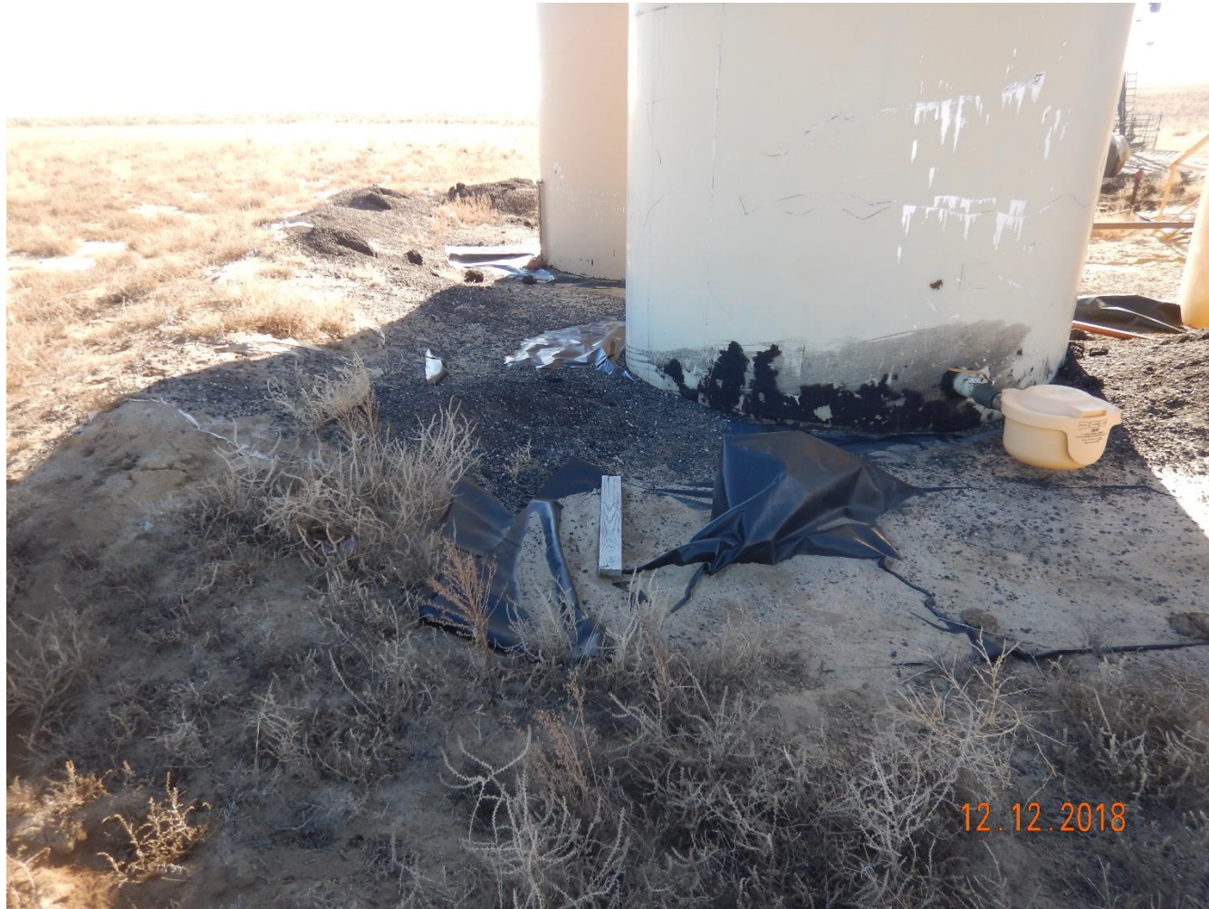
Photo 19: Photo taken from the northeast end of the tanks on location, facing south. Previous inspections documented that the berms around the tanks were inadequate and required operator to repair or install berms, or secondary containment devices. Photo shows berms, or other secondary containment devices have not been repaired or installed; berm missing from the northern end of the tanks.
