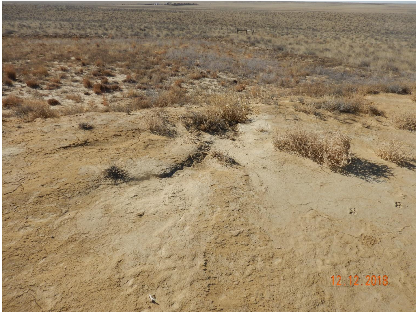
Photo 3: Photo taken from the North end of the location, facing west. Photo shows erosion has continued to degrade access road and location. Unable to find evidence of maintenance, or evidence that the required BMPs have been installed per 1002.f and corrective actions.
