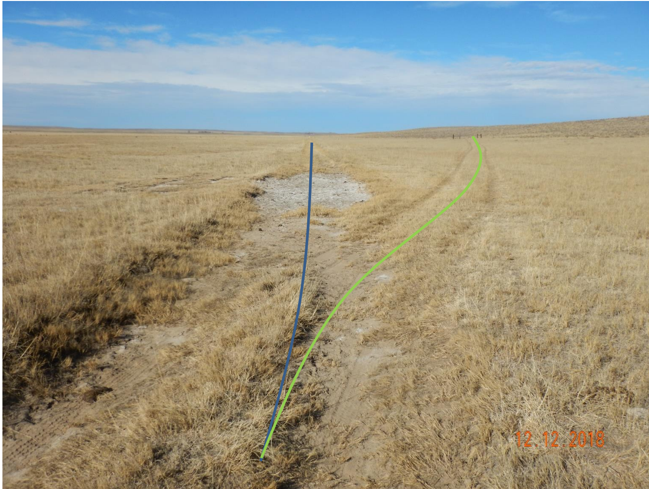
Photo 25: Photo taken from the access road, facing north. Continued from photo 24. Road on the left (blue) is the original access road. Photo shows point where vehicle traffic appears to be traveling off the road (green line) due to a fence without a gate constructed across the access road. Any additional disturbance(s) will require reclamation.
