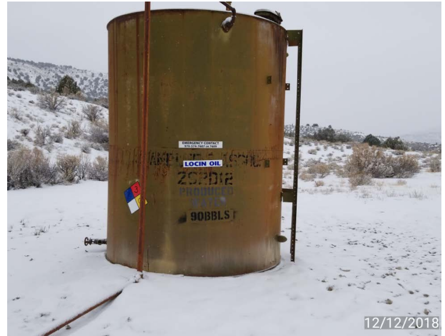
Photo 2. Tank with insufficient berm height.
