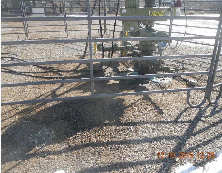
Stained gravel and absorbent wipes near well head.
