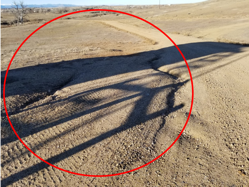
Photo 1. Photo taken from the facility location along the access road, facing North. Appears stormwater runoff is causing rill erosion along the access road between the facility and the drainage to the North.
