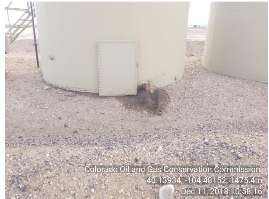
Photo 4 Stained soil under VLV in back of Production tanks
