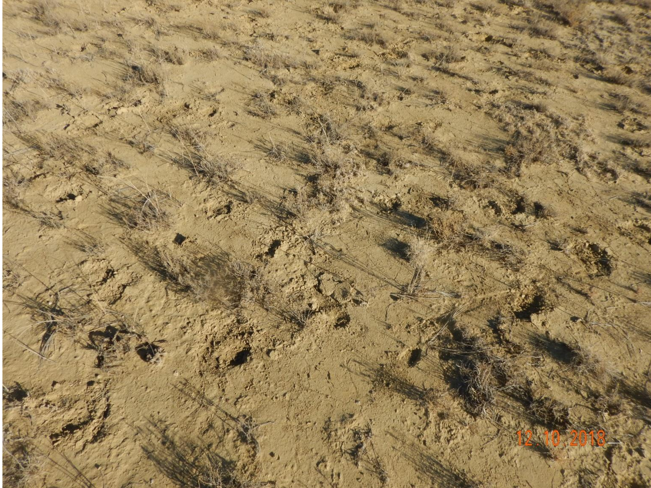
Photo 7: Photo taken from the south end of the pad. Photo shows vegetation has not achieved a uniform establishment in accordance with 1004.a
