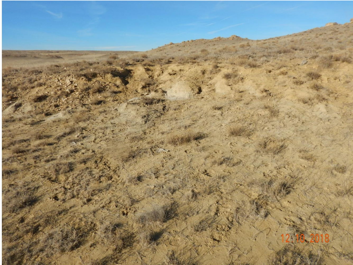
Photo 3: Photo taken from the southwest end of the pad, facing west. Photo shows vegetation has failed to achieve a uniform establishment, and stormwater runoff has caused erosion degradation on the pad.
