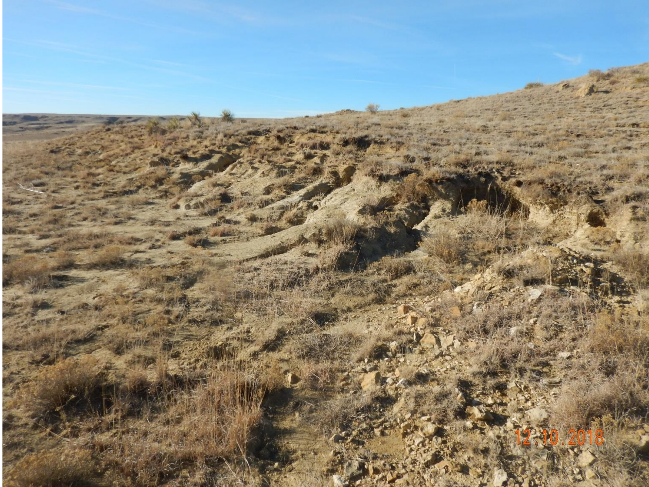
Photo 6: Photo taken from the northwest end of the pad, facing southwest. Photo shows vegetation has failed to achieve a uniform establishment, and stormwater runoff has caused erosion degradation on the pad.
