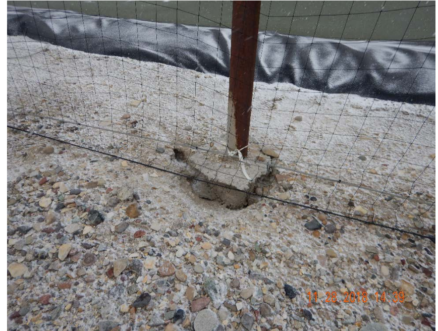
Photo #4 – Maintenance required at several netting posts along west side of pit (1).
