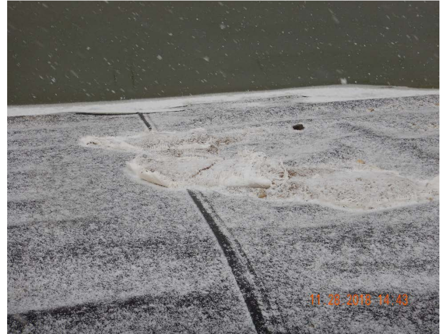
Photo #8 – Foreign material (sand bag remnants) on top of liner on east side of pit.
