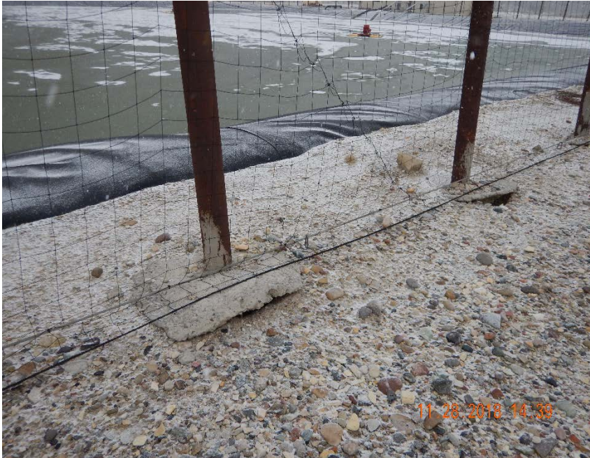
Photo #5 - Maintenance required at several netting posts along west side of pit (2).
