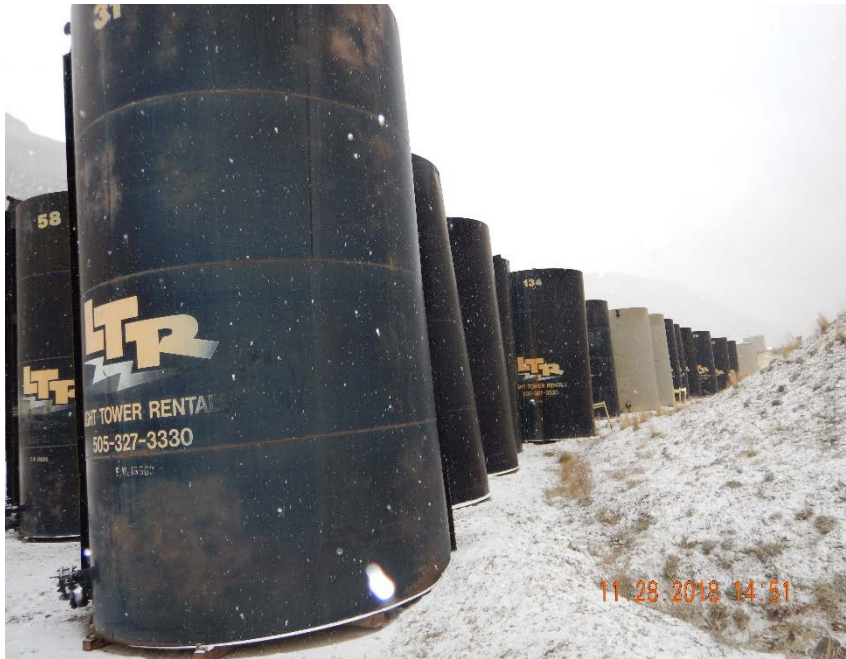
Photo #11 – View of south tank battery from SE corner. Note absence of earthen berm along east side of tank battery.
