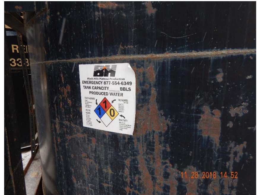
Photo #12 – One of several tanks in south tank battery that was labelled “Produced Water.” These tanks did not appear to be in use on inspection date, many were labelled “Do not use”.
