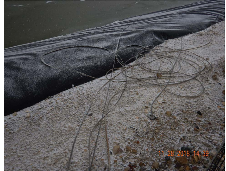
Photo #6 – Unused equipment (steel cable) stored on west side of pit, in contact with pit liner.
