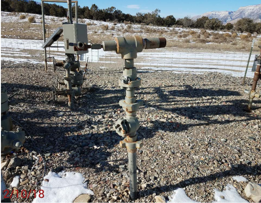
Location Photo #3, unmarked flow line riser.
