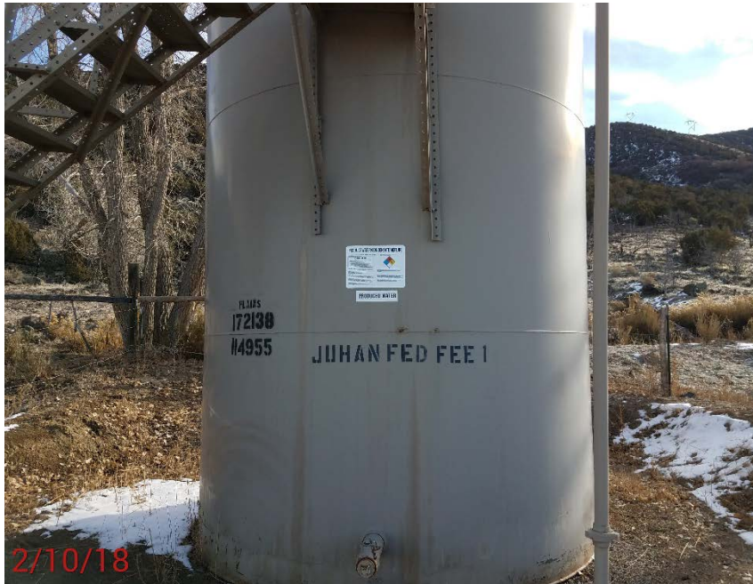
Location Photo #5, Tank Missing capacity information.
