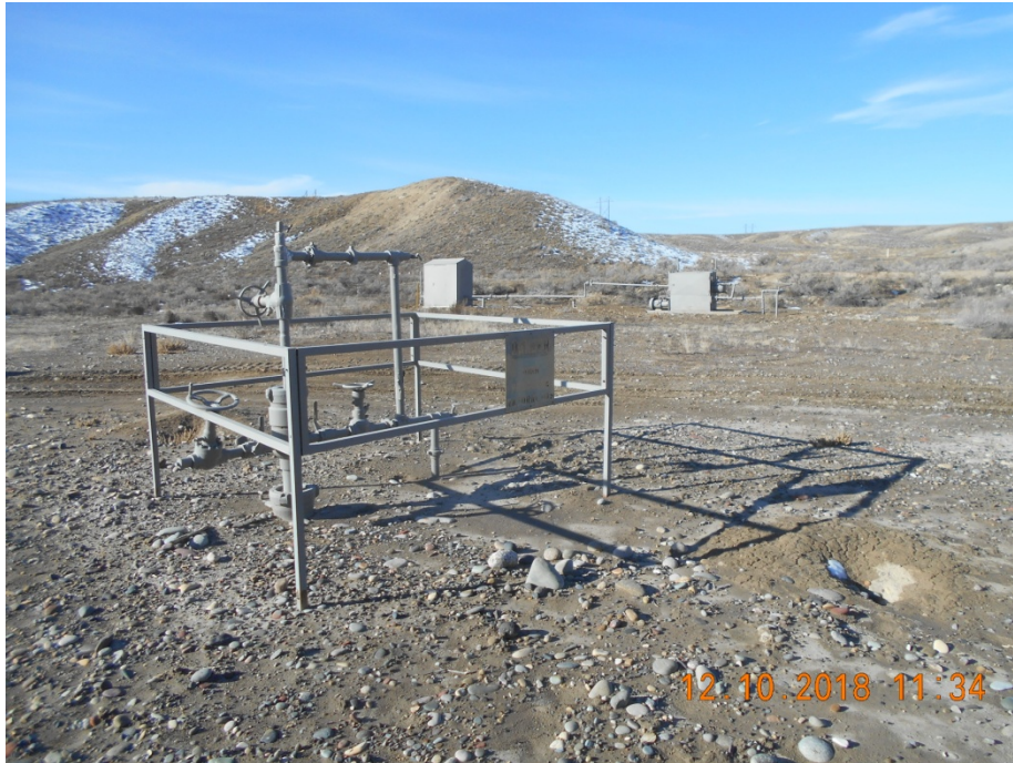
Wellhead with fencing and missing sign
