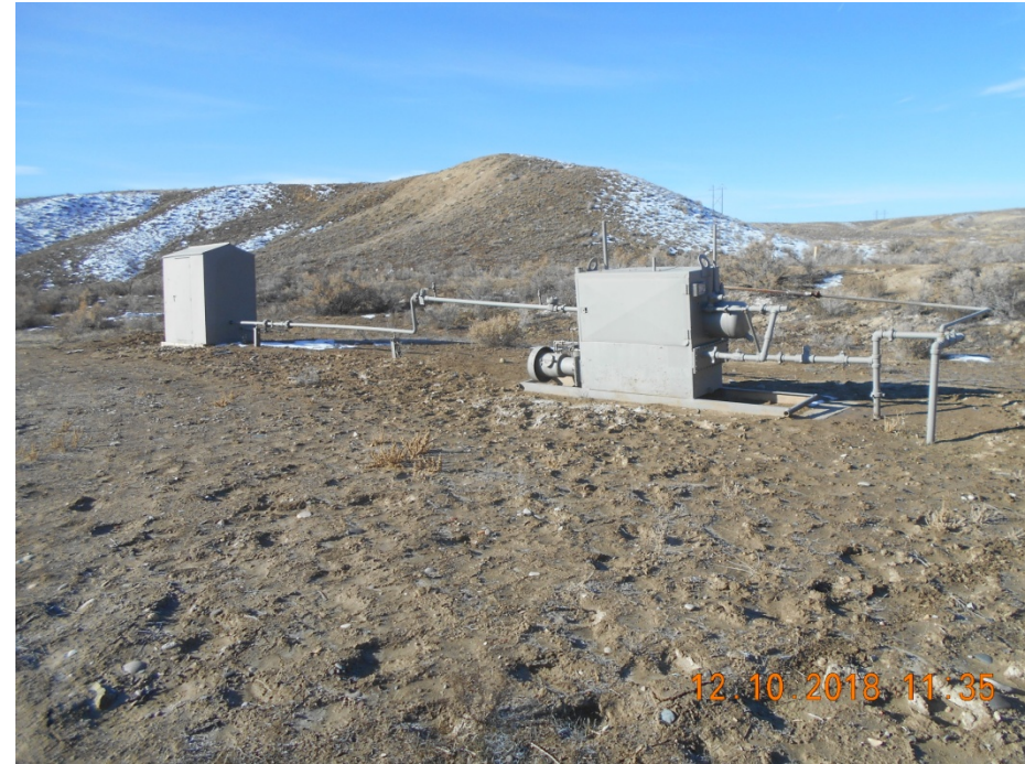
Separator and Meter housing
