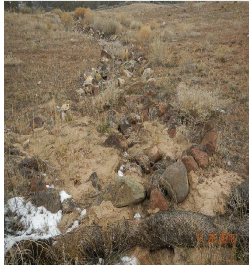
Photo#12: Undercutting of rocked drain and wattles.
