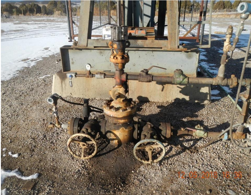
Stained soil at #4-1 well head.
