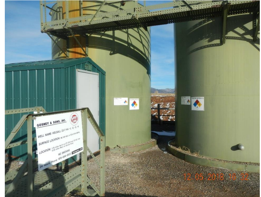
2 - 300 bbl. produced water ASTs.
