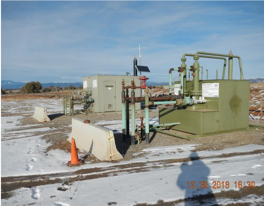
Horizontal heated separators for wells #4-1 through #4-4.
