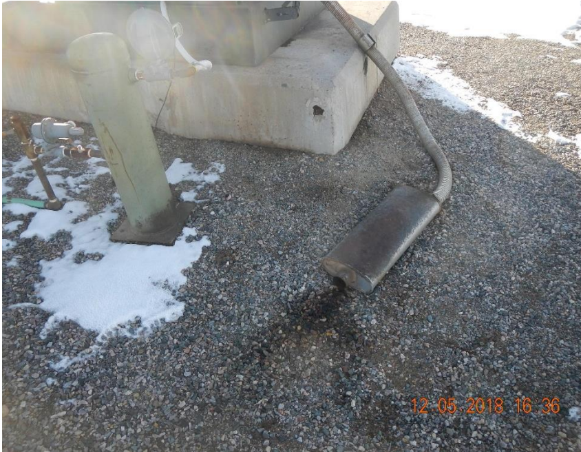
Stained soil at exhaust for prime mover.
