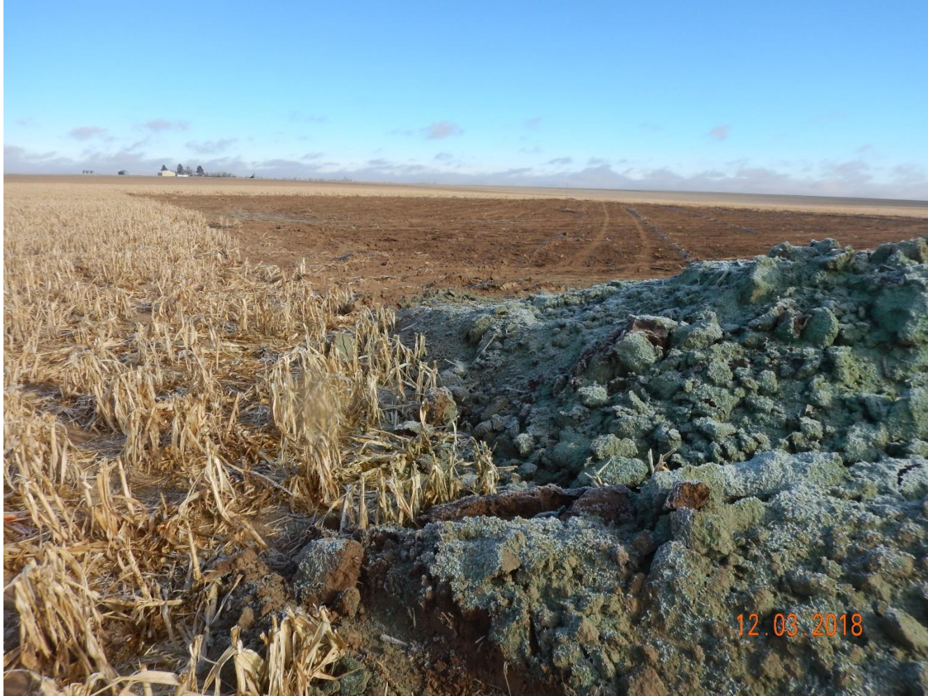
Photo 11: Photo taken from the southwest corner of the pad, facing northeast. Photo shows that no perimeter stormwater controls appear to have been implemented on the west end of the location.
