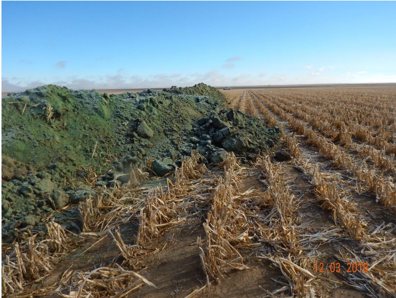
Photo 12: Photo taken from the southwest corner of the pad, facing northeast. Photo shows that hydromulch appears to have been applied to the soil stockpile. Additionally, it does not appear that perimeter stormwater controls were implemented, and/or existed prior to hydromulch, on the south end of the location.
