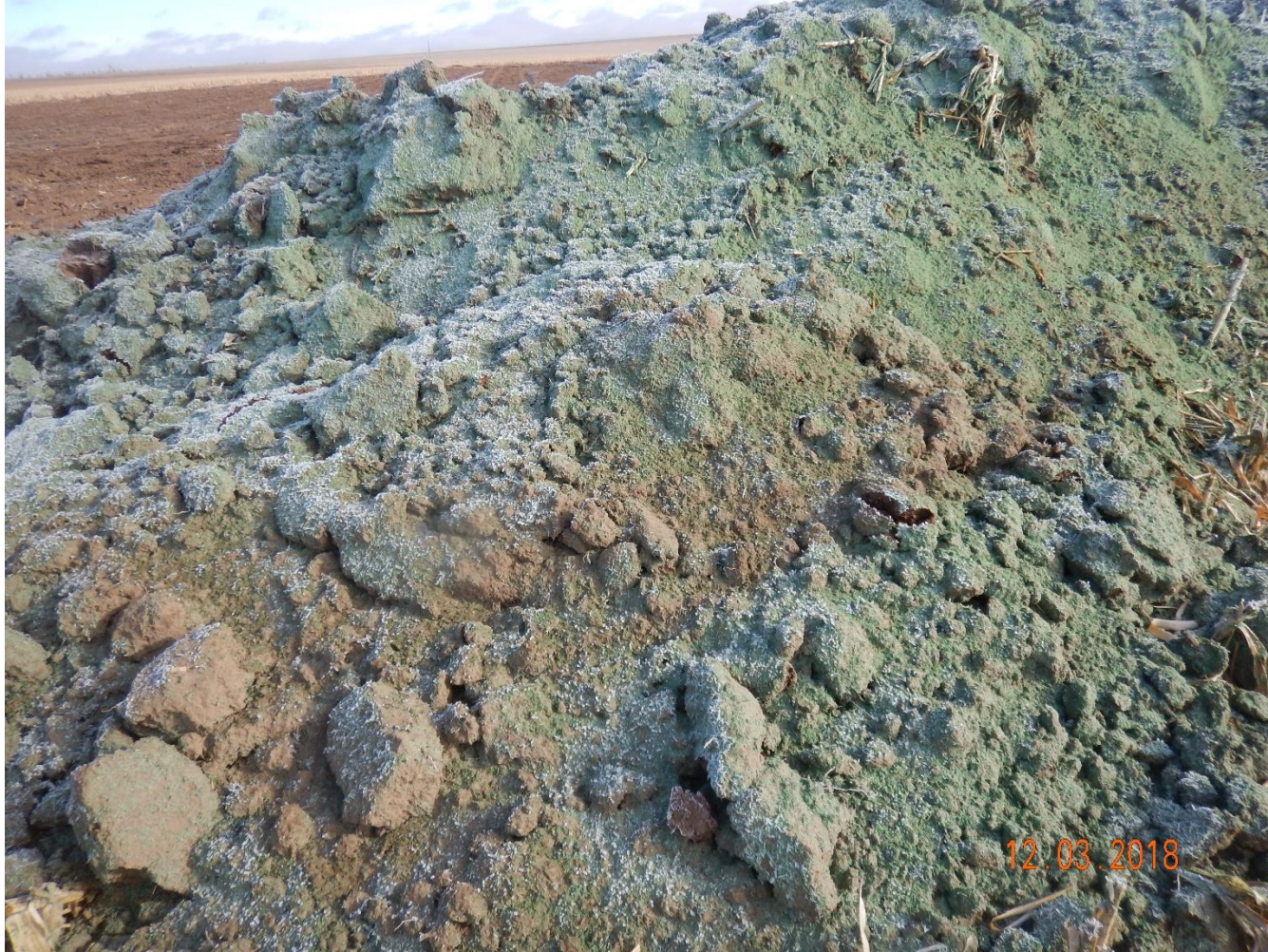
Photo 13: Photo of hydromulch applied to soil stockpile.
