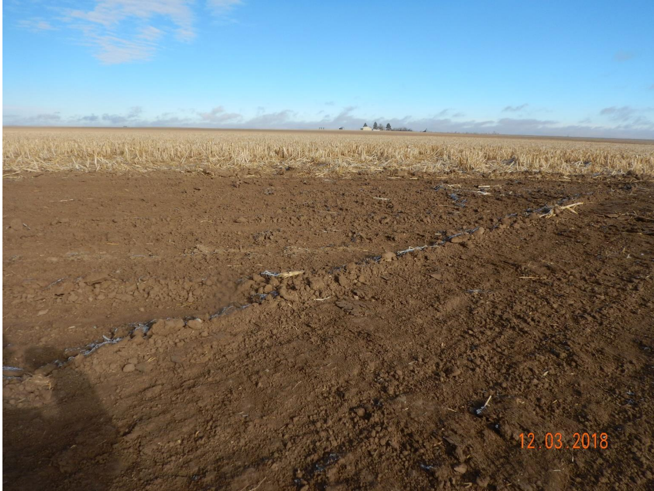
Photo 16: Photo taken from the center of the pad, facing North. Photo shows areas of the south and west end of the pad where ~1 inch of soil appears to have been salvaged when compared to the adjacent reference.
