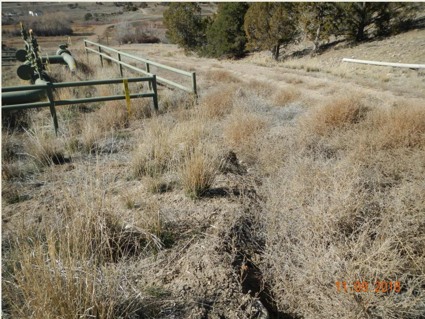
Photo 5. View of erosional channeling occurring within the western project area.
