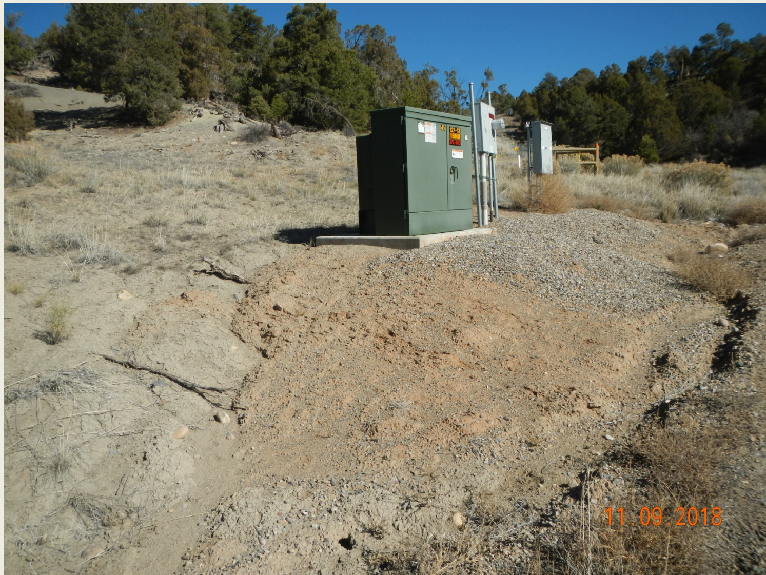
Photo 5. View of erosional channel approximately 1.5 feet wide and 10 inches deep, forming within the northern project area around project facilities.
