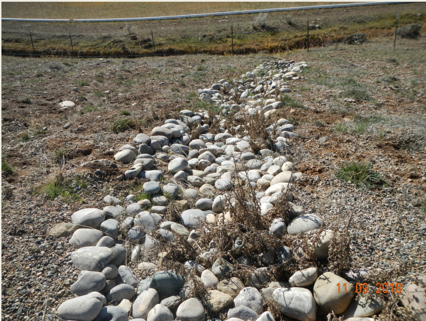
Photo 5. View of cobble rundown in the southwestern project area appears to be functioning at this time, but may soon require maintenance. Approximately 500 Canada thistles (visible in the cobble in the foreground) are growing within the southern interim reclamation areas.
