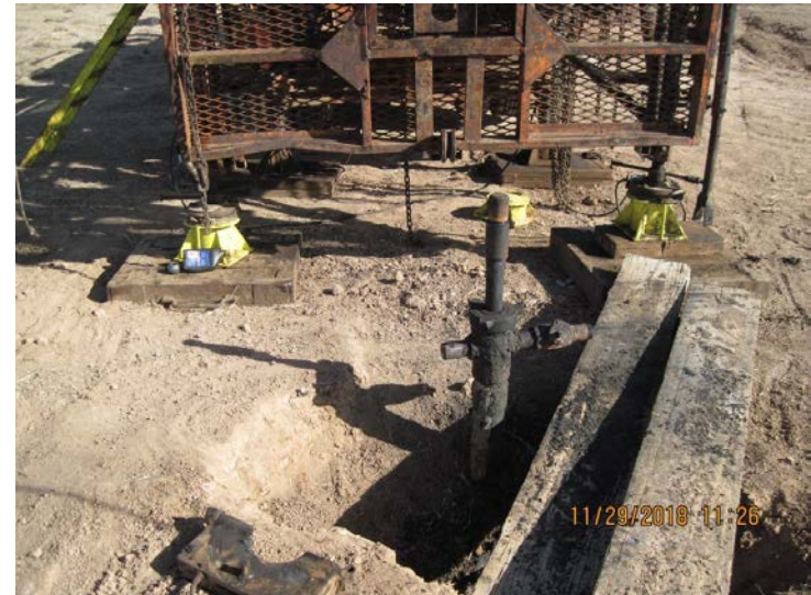
6. Wellhead dug out
