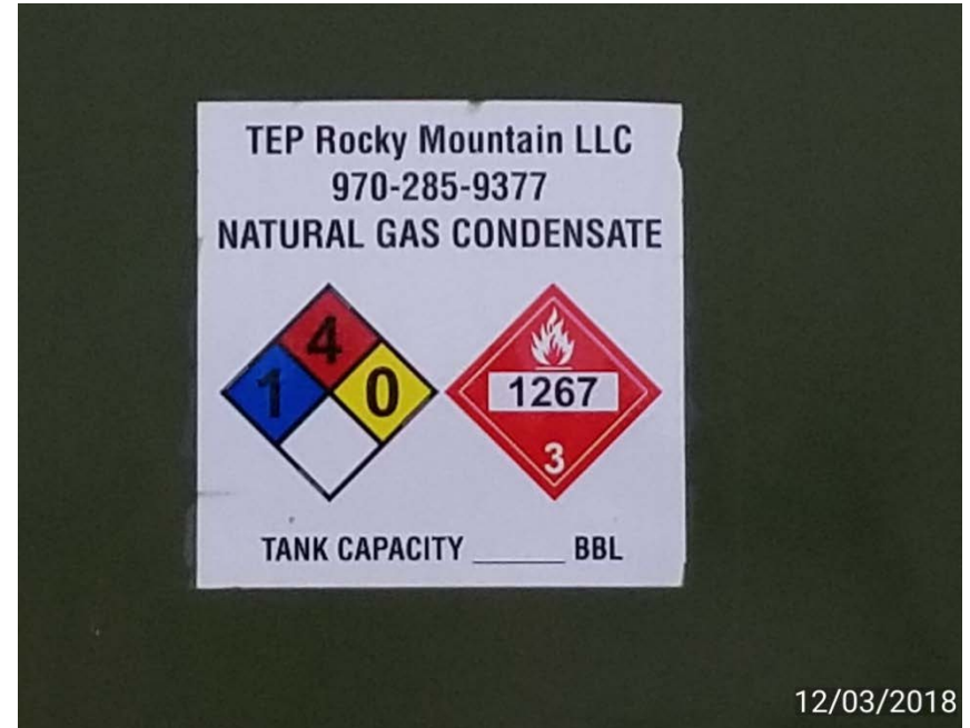
Photo 2. Tank capacity of 210 BBL missing.
